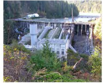
Elwha Dam Port Angeles, WA
