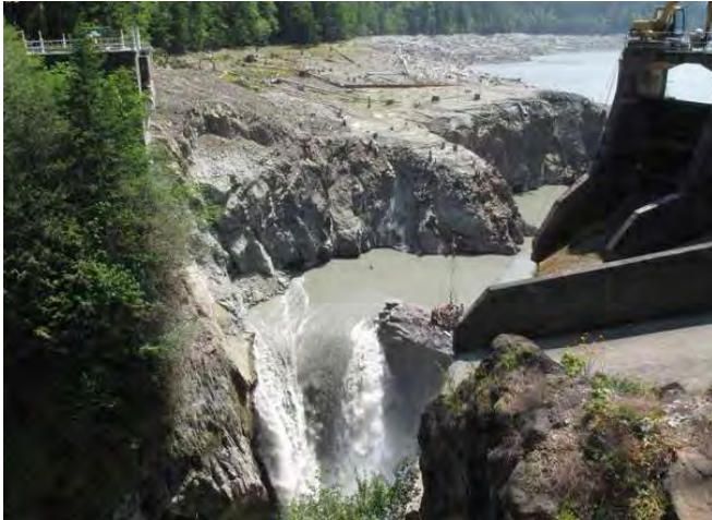
Glines Canyon dam removal
