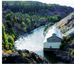
Klamath Hydroelectric Project Humboldt County, CA
