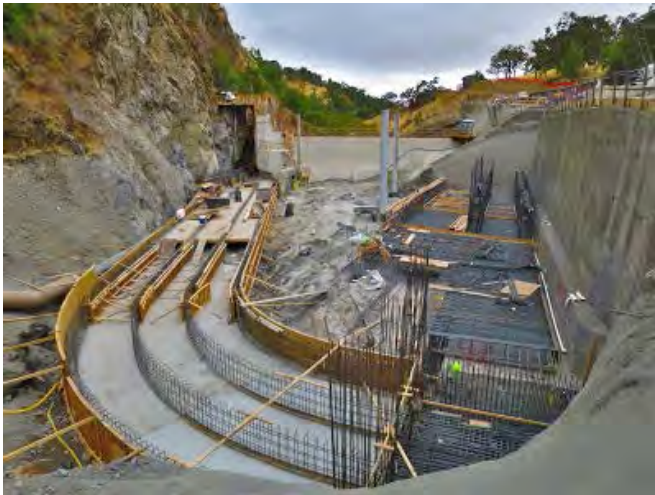
Alameda Creek Diversion Dam Fish Passage Facilities under construction, 2016
