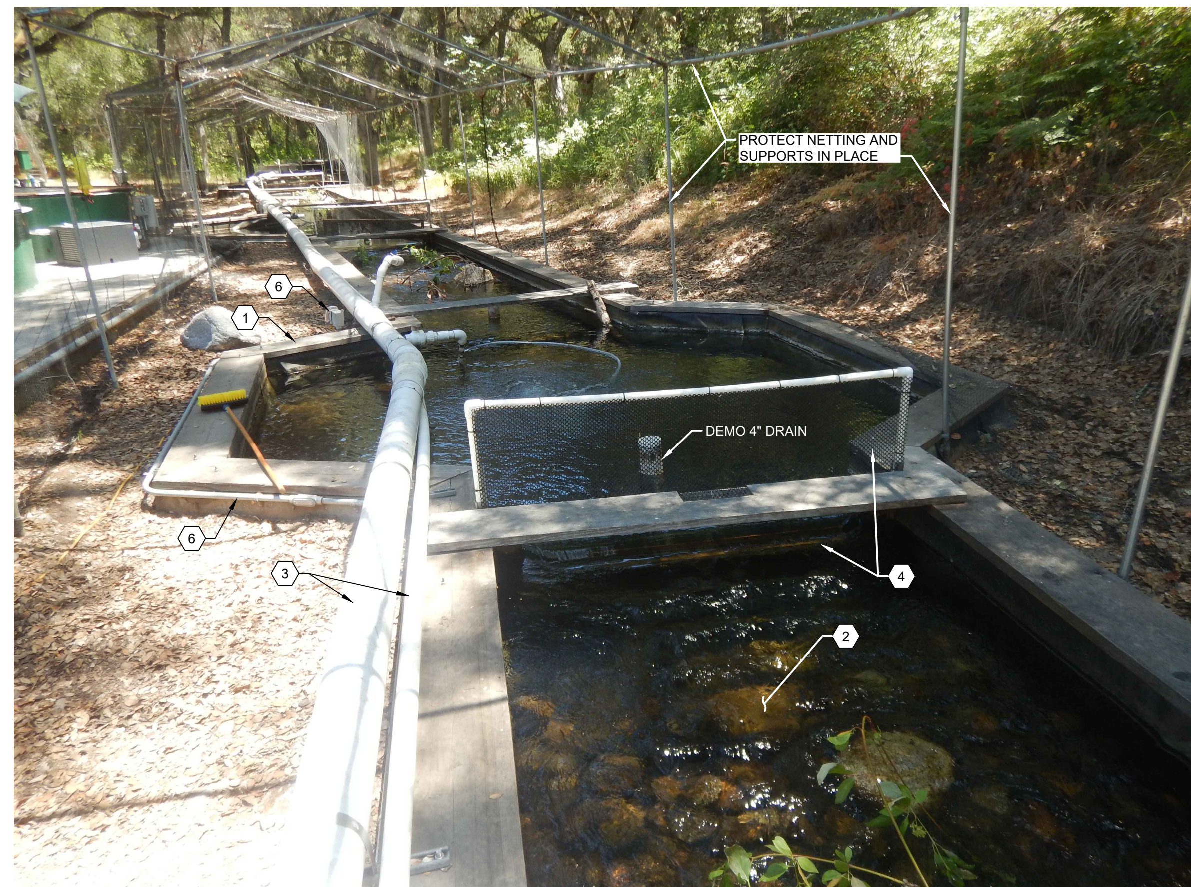
3 EXISTING POOL PHOTO NO SCALE
