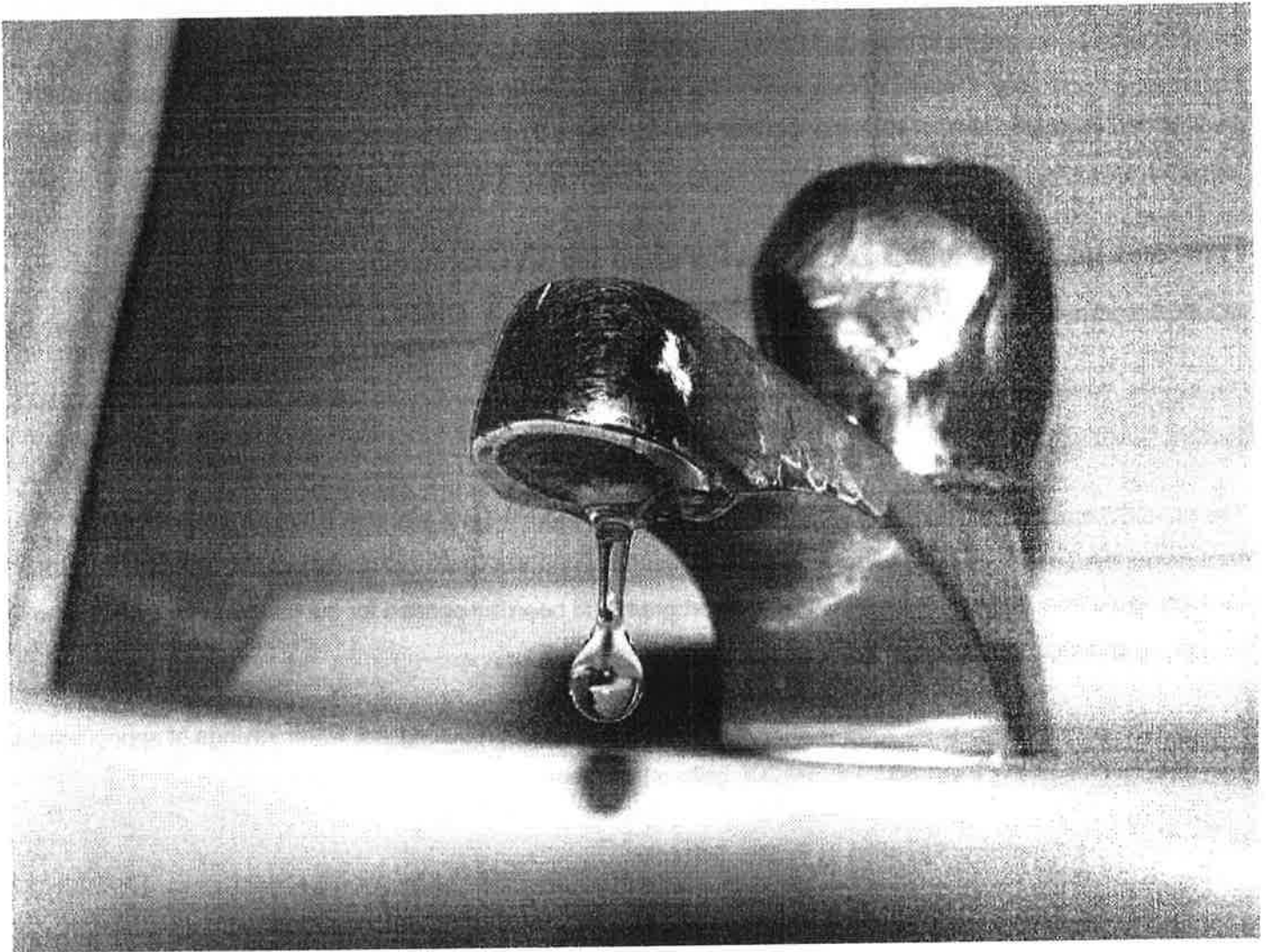
Soquel Elementary, and New Brighton Middle School - toilets and faucets
