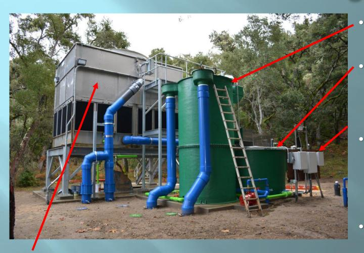
Elevated cooling tower eliminates repumping
