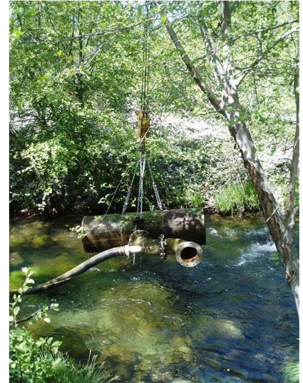
Existing pumps are located next to the river deep inside a concrete caisson (above and left) that is inaccessible at high flows. The existing drum screen (at right) is subject to clogging from silt, sand, and debris.
