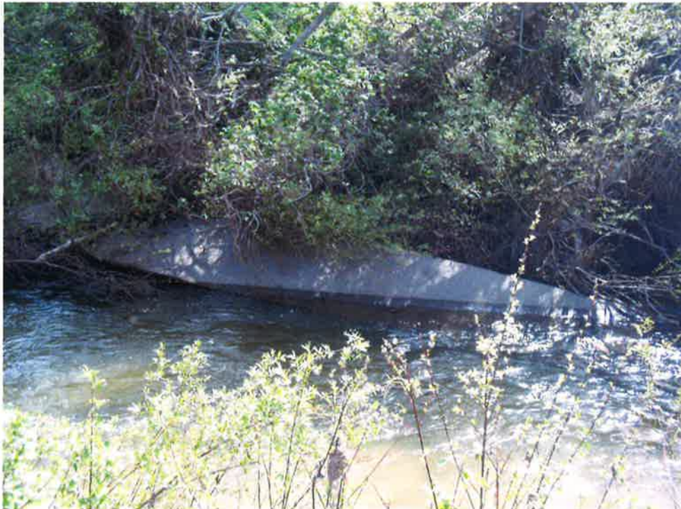
Concrete Bridge Deck during higher flows in March 2017
