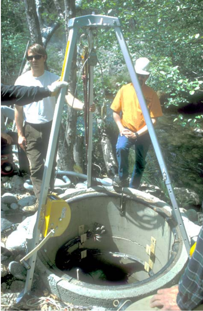
Left - existing caisson/wet well adjacent to Carmel River at the Sleepy Hollow Steelhead Rearing Facility. Drum screen in channel is in middle right background (under cobbles).
