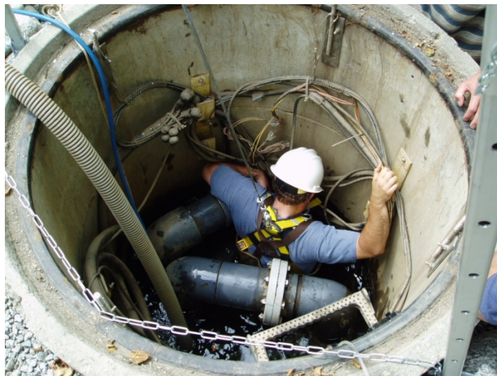
Below - Looking into existing pump enclosure
