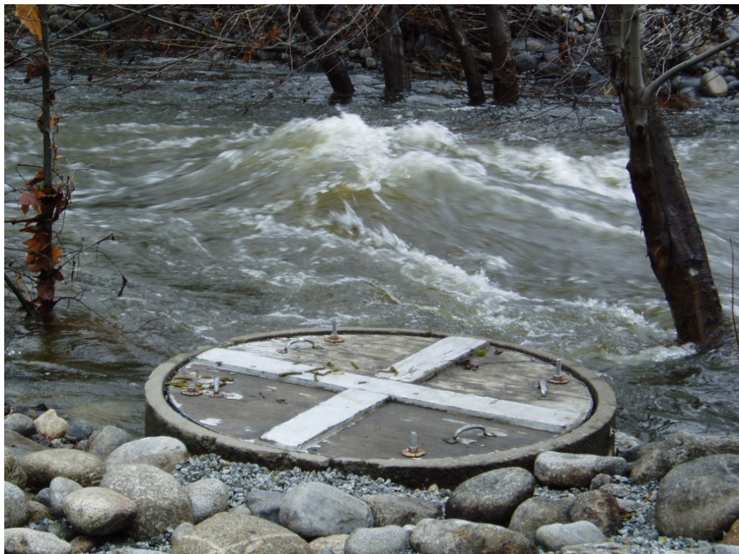
Below – winter flow at screen and pump enclosure
