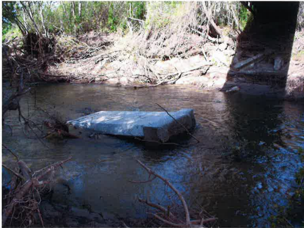
Concrete Bridge Pier during higher flows in March 2017
