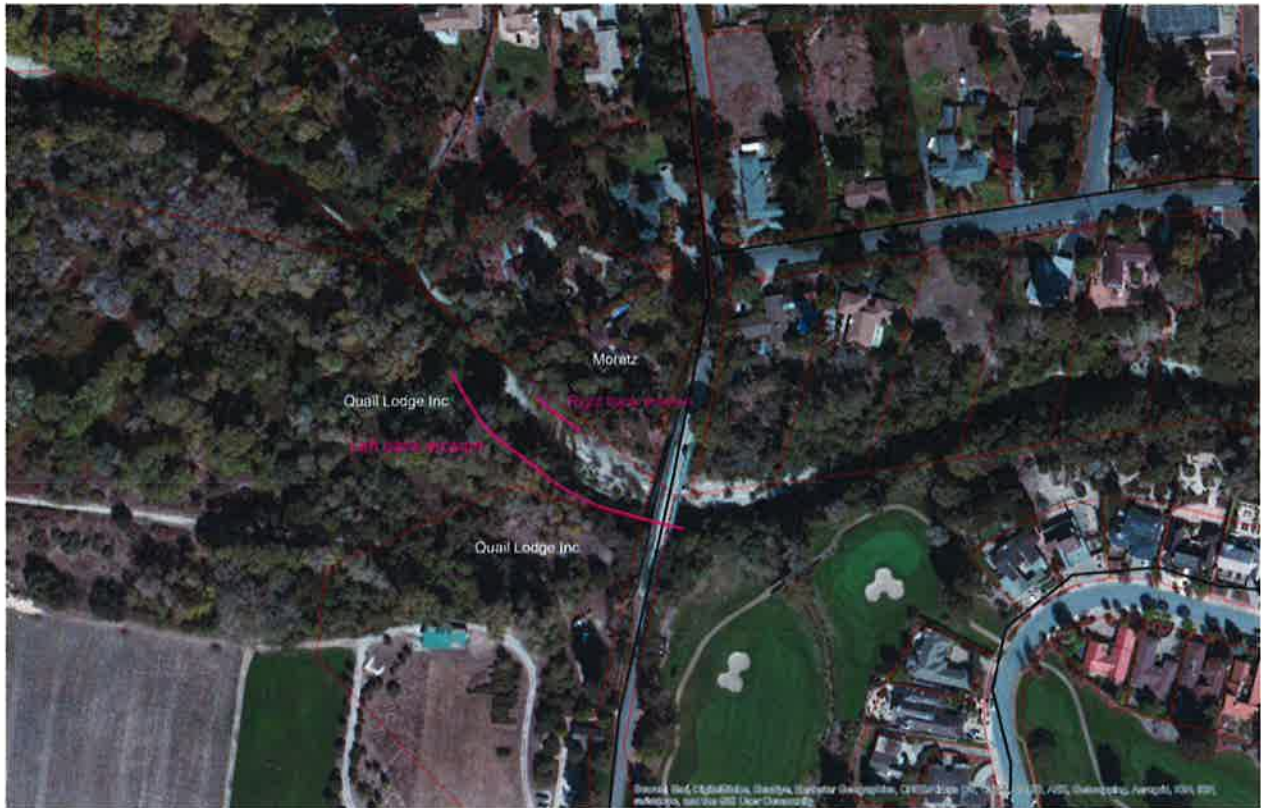
Aerial Image showing locations of erosion just downstream of Rancho San Carlos Rd. Bridge
