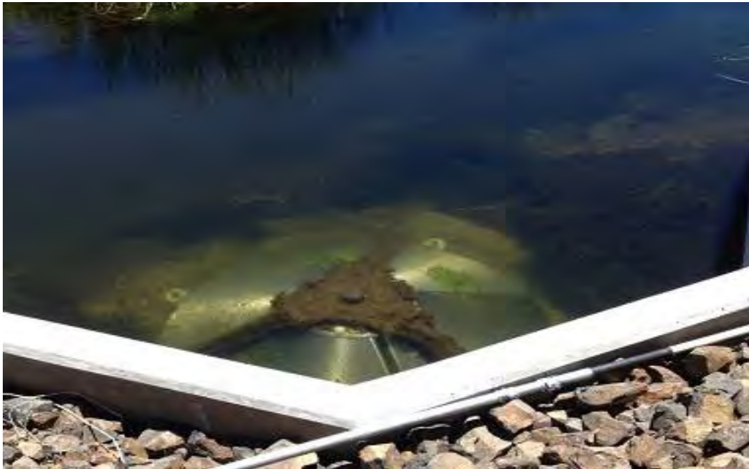
Image 2- Example of cone screen underwater in an alcove with external cleaning brushes in operation.
