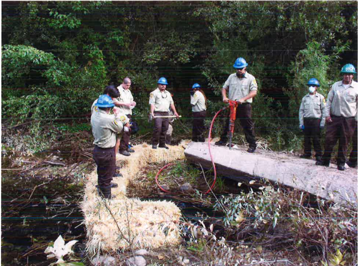
Example of concrete pier removal that was carried out in 2008.
