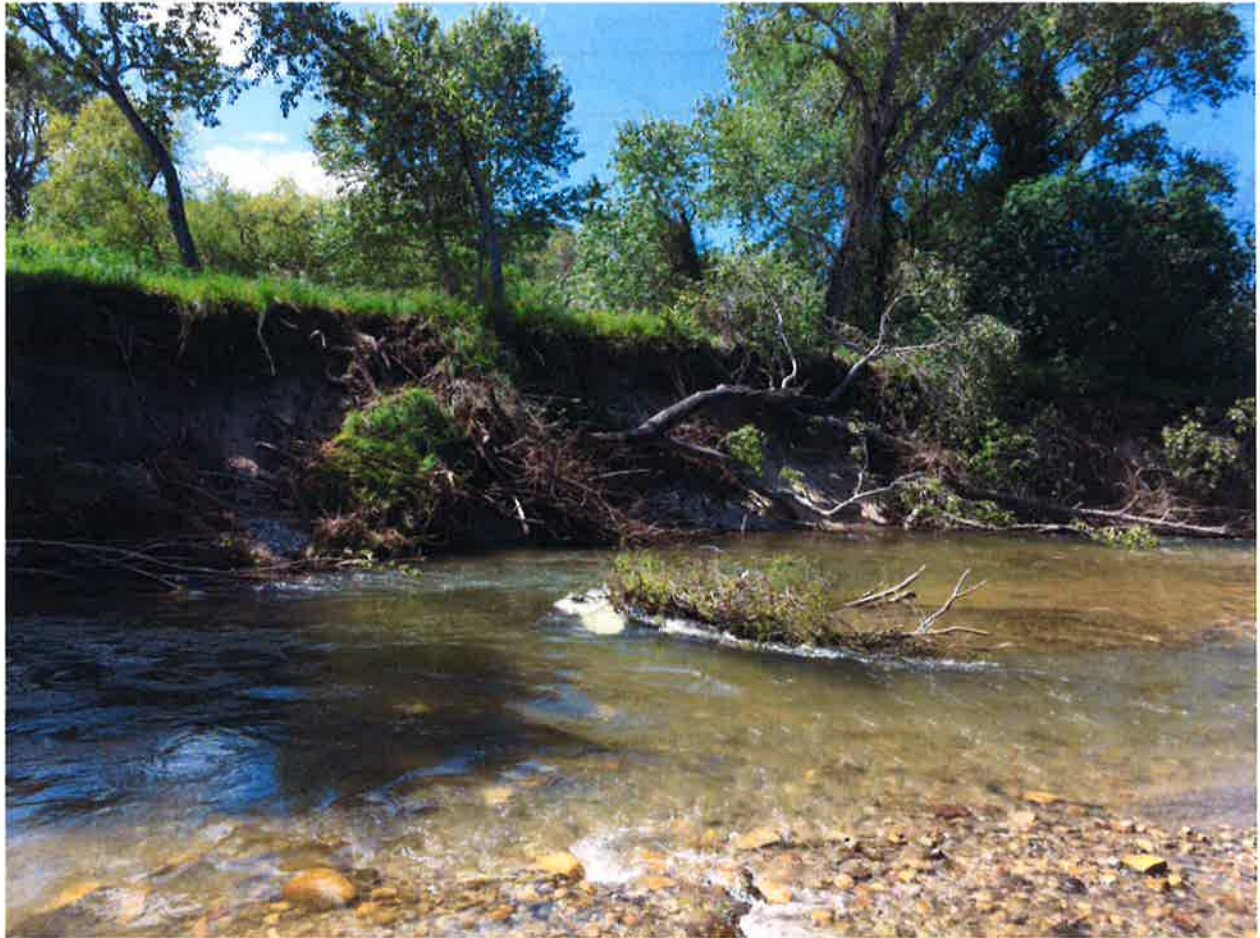
Left bank erosion on outside of meander bend with mature cottonwood forest trees dropping into river during high flows along the Quail Lodge Inc. property, Carmel River, Monterey County, California, March 27, 2017.
