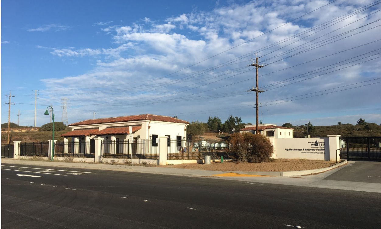
Figure 5 Santa Margarita Facility from the South
