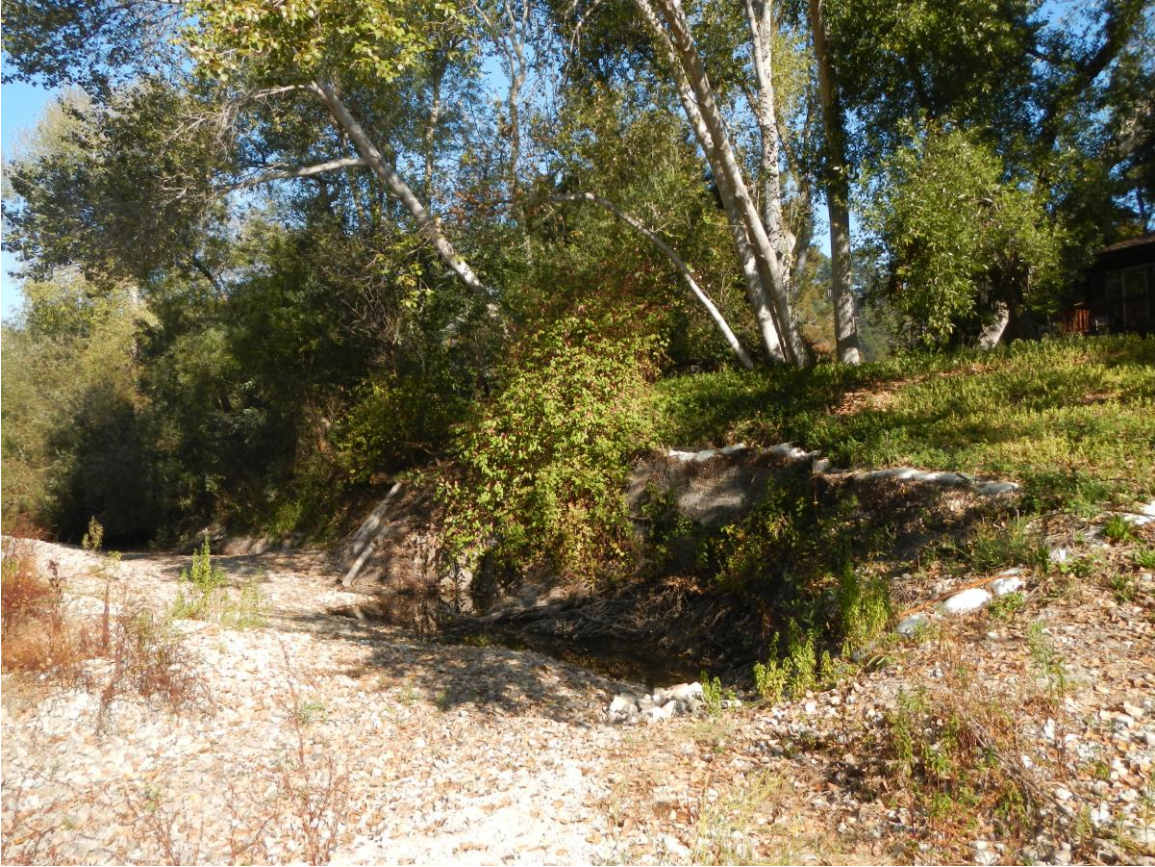
Photo looking downstream at erosion along Big Sur Land Trust/ Lake and Asselborn properties, Carmel River, Monterey County, California, November 7, 2011.
