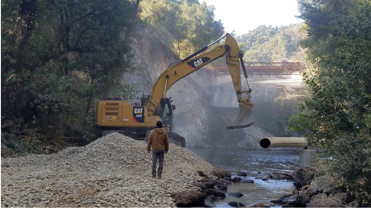
Placing the gravel at the Los Padres Dam plunge pool. Winter river flows will move the gravel downstream into the preferred spawning habitat. September 2019.
