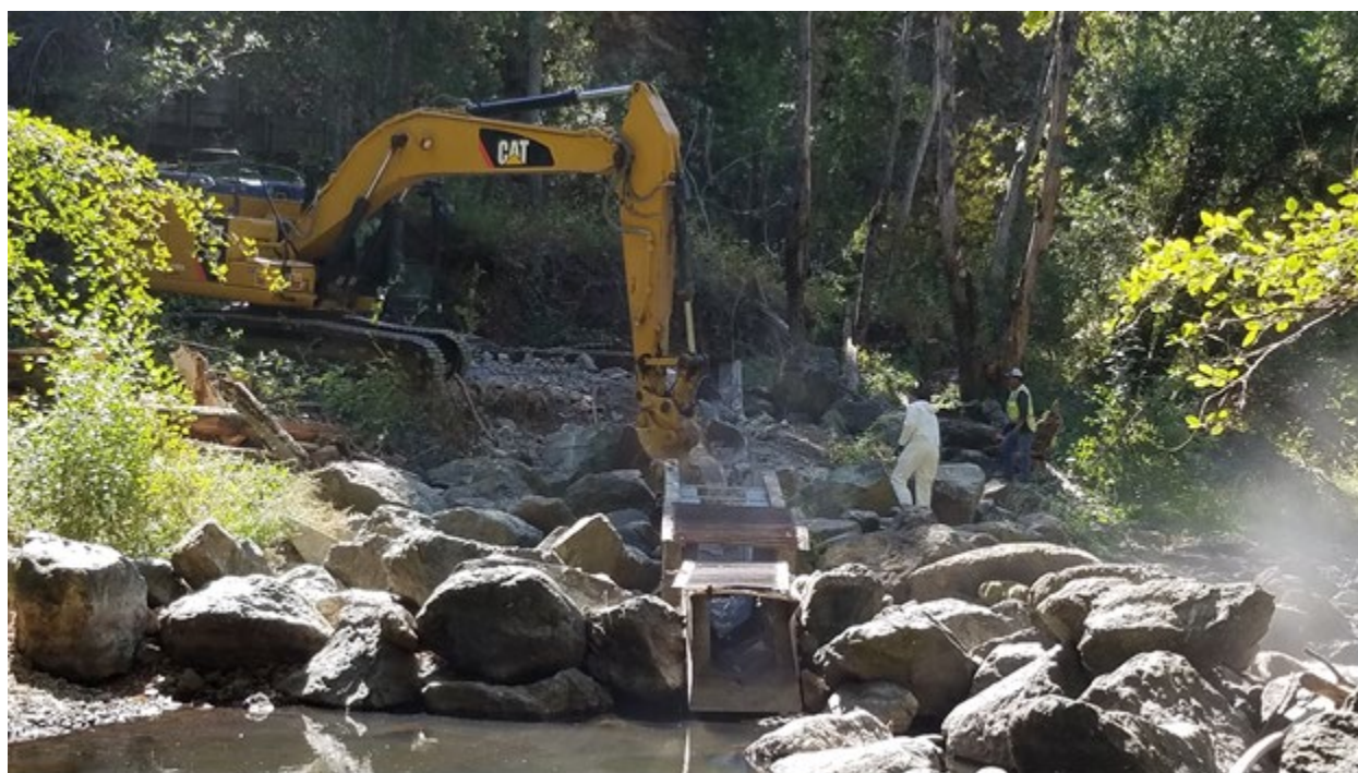
Removal of the old abandoned fish trap/ladder and boulders at Los Padres Dam as part of the spawning gravel augmentation project, September 2019.
