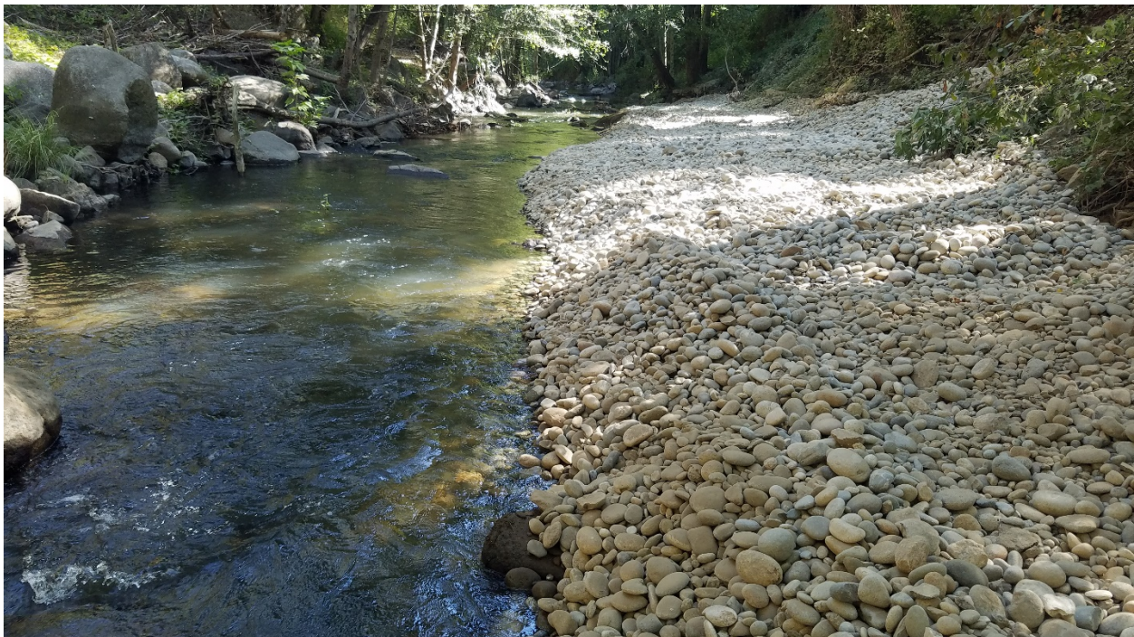
Spawning gravel placed along the river bank below Los Padres Dam. Winter river flows will move the gravel downstream into the preferred spawning habitat. September 2019.
