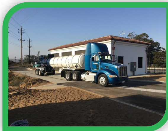
Construction of Santa Margarita Water Treatment Facility was completed in 2020
