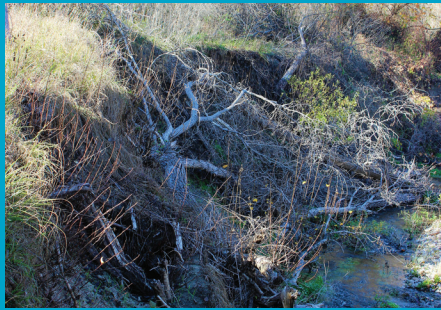
Cultural and Historic Streambank Threatened by Storm Erosion
