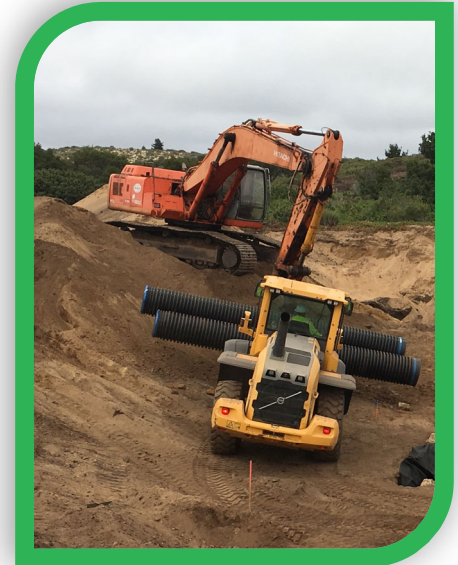
Construction of expanded percolation pond to accommodate waters from two additional ASR wells that will enable recovery of ASR and Pure Water Monterey stored waters.
