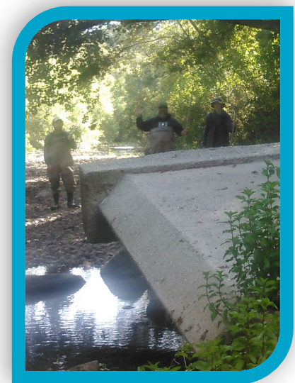
Concrete bridge pier and deck lying in the Carmel River before removal by staff
