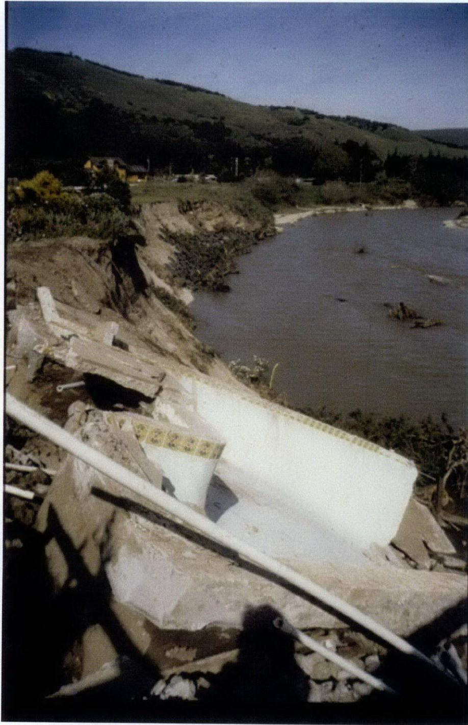
Above – ca spring 1982 – looking upstream along the Carmel River, near River Mile 6 at the remains of a back yard pool that was undermined. Note the use of car tires for streambanks protection (middle background).
