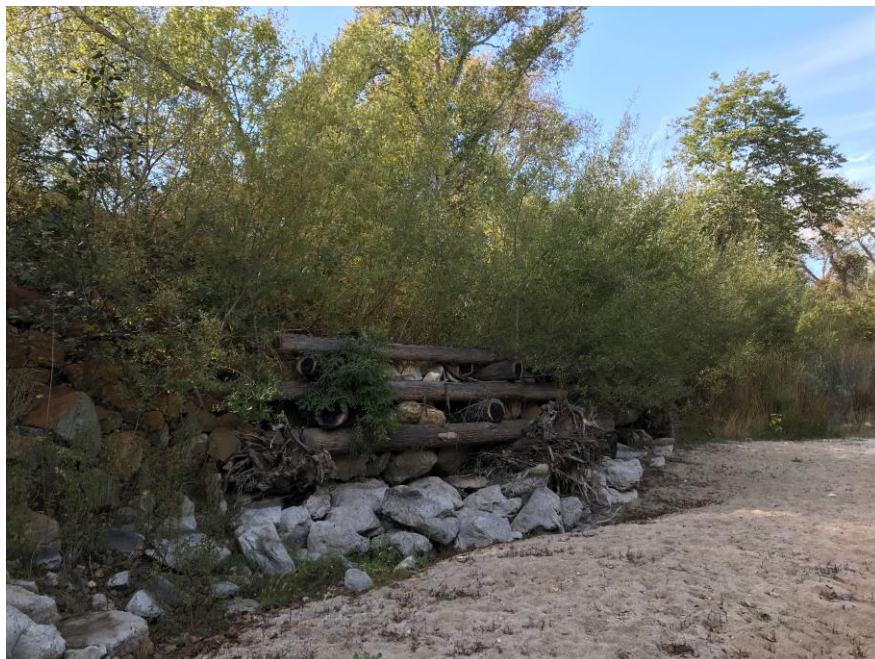
Left Bank Looking Downstream after Bank Stabilization (October 2022)
