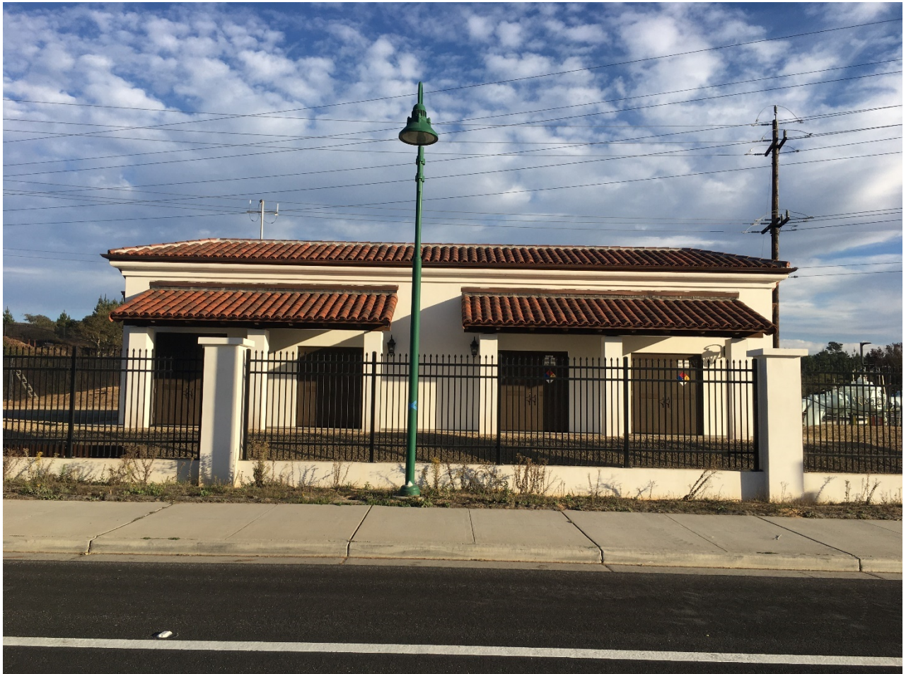
(Photo: ASR Chemical Building)
