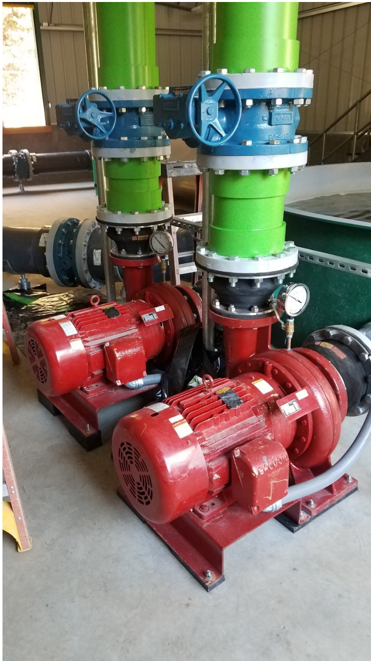
(Photo: Sleepy Hollow Facility Pumps)
