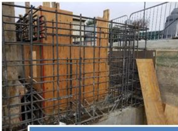
Diversion Structure #2 Rebar and concrete forms
