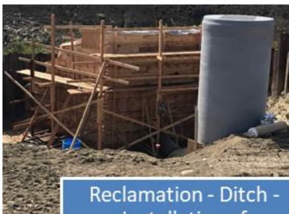
Reclamation - Ditch - Installation of Trash Rack & Fish Screen
