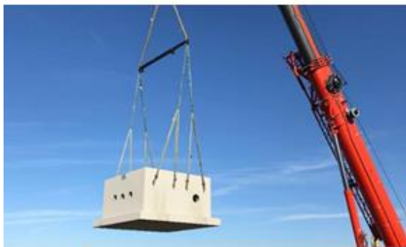
Reclamation - Ditch - Setting PS Valve Vault
