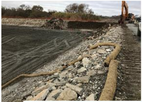
Stormwater BMP's, removing rip-rap
