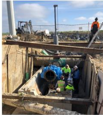
Nearly Completed Hot-tap Valve Vault
