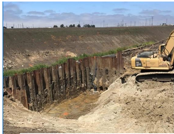
Pump Station Excavation in Shoring Box
