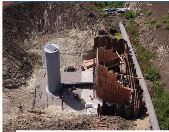
Weir manhole, Sidewall Form Rebar
