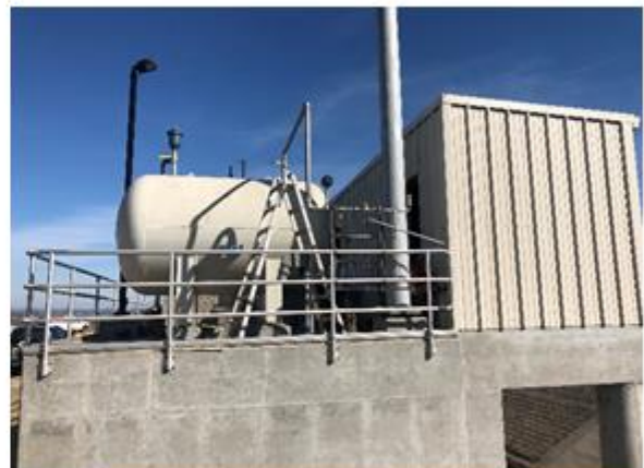
Surge Tank Appurtenant Installation
