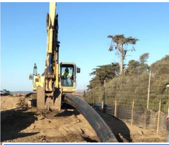
HDD Pull Back Operations
