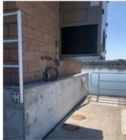
HVAC System installed and conduit stub-outs for Water Quality Analyzer Cabinet
