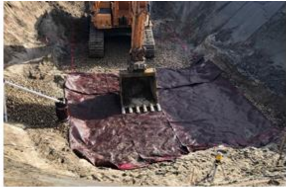
Placing concrete slurry subgrade for Pump Station wet well
