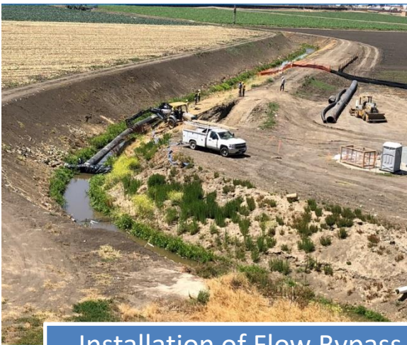
Installation of Flow Bypass
