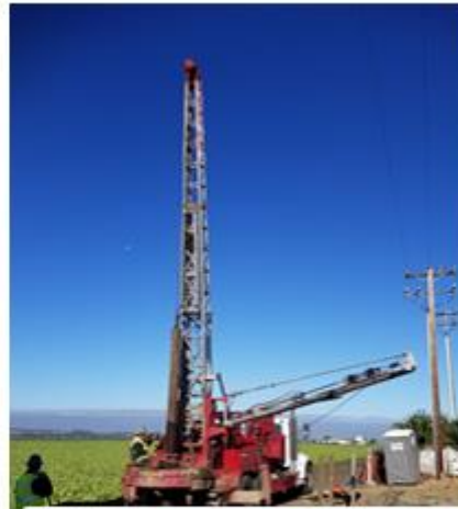
Drilling Dewatering Wells
