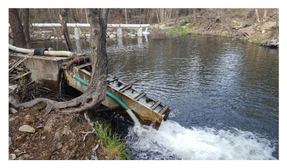
Figure 2-8 Denil Type Fish Ladder and Auxiliary Water Supply Pipe Below Los Padres Dam
