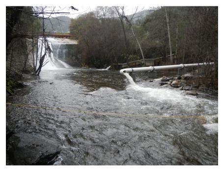
Figure 2-11 Fish Bypass Outfall Downstream of Spillway Plunge Pool and Fish Ladder
