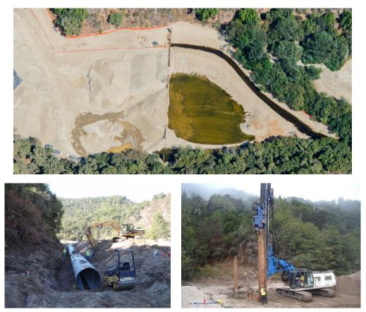
Figure 5-5 San Clemente Dam Removal Upstream Diversion Structure and Diversion Pipe; Bottom Two Installation Photographs, October 2013; Top Operating Photograph, August 2015
