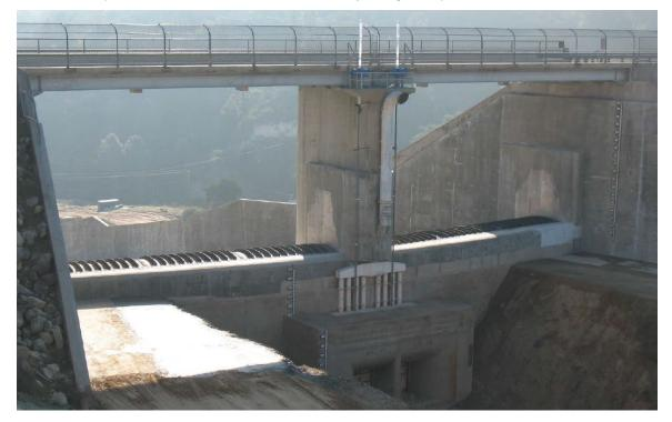
Figure 5-16 Pneumatically Actuated Spillway Gate at Nacimiento Dam (Gates Down – Post-Construction)
