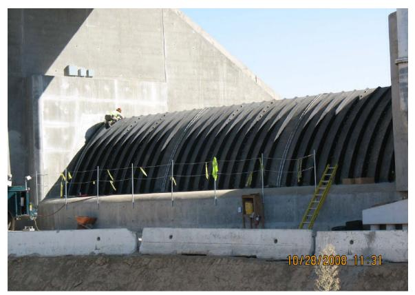
Figure 5-14 Pneumatically Actuated Spillway Gate at Nacimiento Dam (Construction – from Upstream Reservoir Side)
