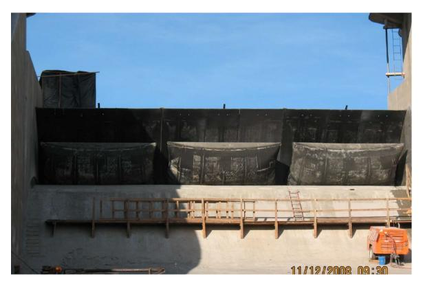
Figure 5-15 Pneumatically Actuated Spillway Gate at Nacimiento Dam (Construction – from Downstream Spillway Side)
