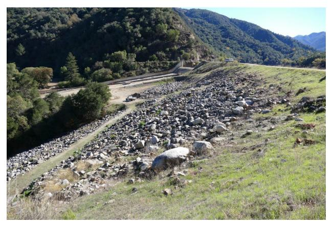
Figure 2-3 Downstream Face of the LPD Embankment
