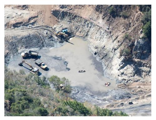
Figure 5-6 Sediment Excavation of Lower Reservoir Sediments, San Clemente Dam Removal, July 2014
