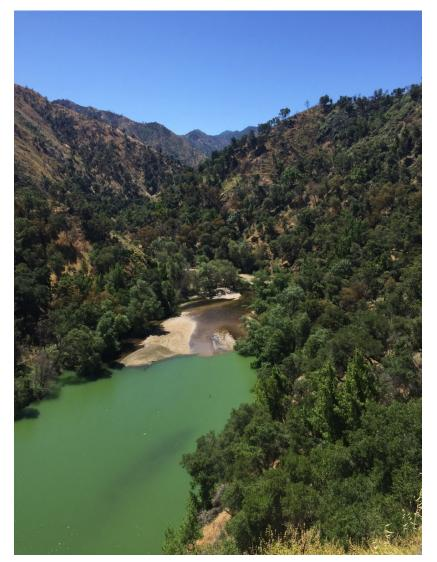
Figure 2-21 Photograph Showing Sediment Delta Encroachment on Reservoir Pool, 2017
