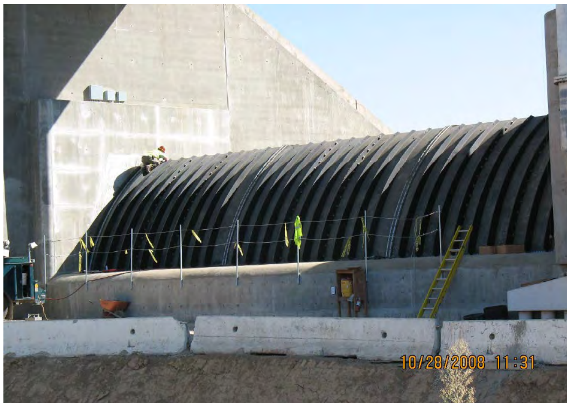
Figure 22 Pneumatically Actuated Spillway Gate at Nacimiento Dam (Construction – from Upstream Reservoir Side)
