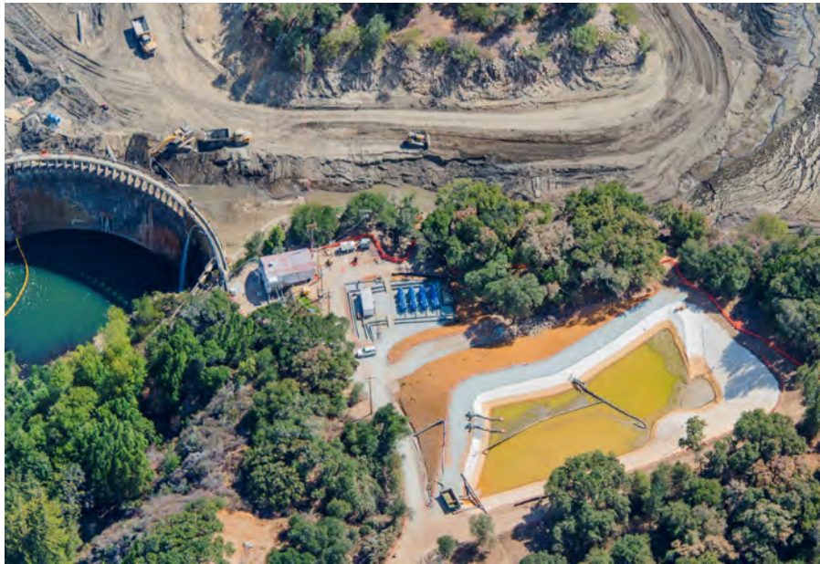
Figure 15 Dewatering Treatment System and Basin, San Clemente Dam Removal, August 2015
