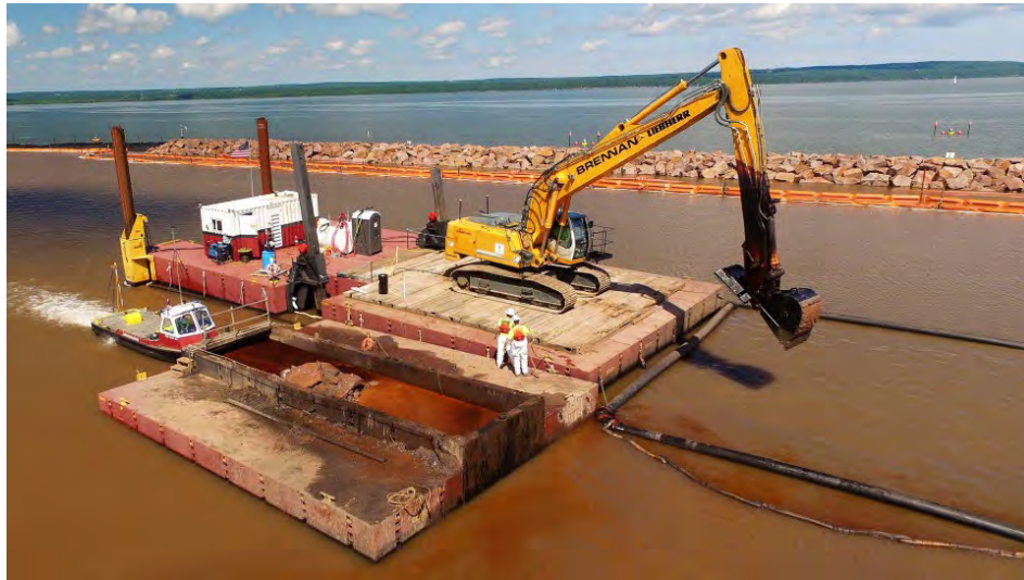
Figure 28 Conventional Excavator on Flexi-Float Barge
