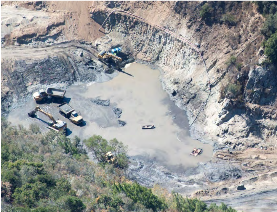
Figure 18 Sediment Excavation of Lower Reservoir Sediments, San Clemente Dam Removal, July 2014
