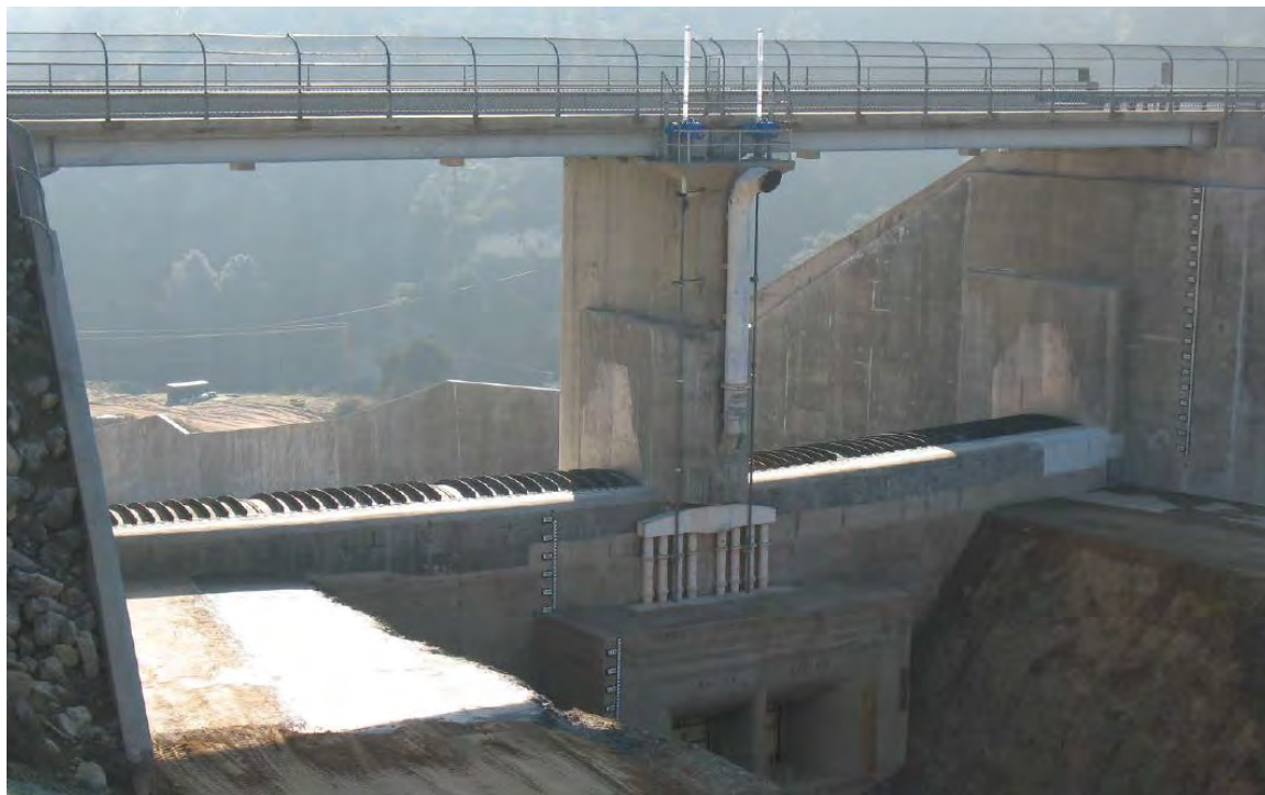
Figure 24 Pneumatically Actuated Spillway Gate at Nacimiento Dam (Gates Down – Post-Construction)
