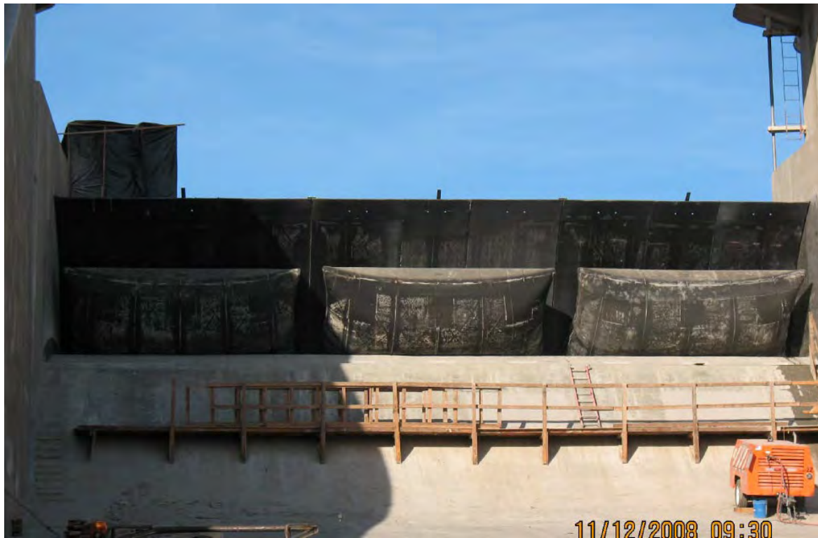
Figure 23 Pneumatically Actuated Spillway Gate at Nacimiento Dam (Construction – from Downstream Spillway Side)
