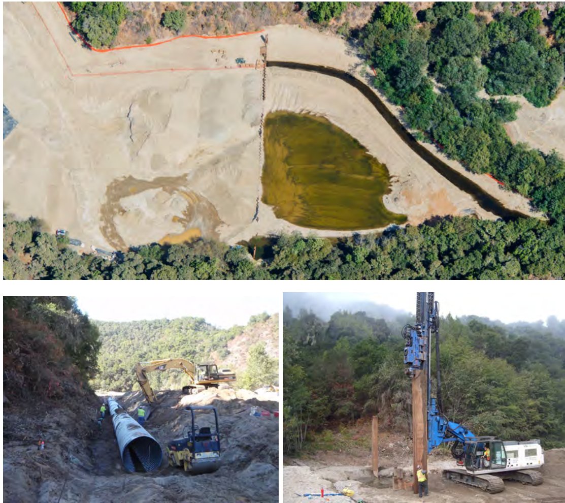
Figure 17 San Clemente Dam Removal Upstream Diversion Structure and Diversion Pipe; Bottom Two Installation Photographs, October 2013; Top Operating Photograph, August 2015
