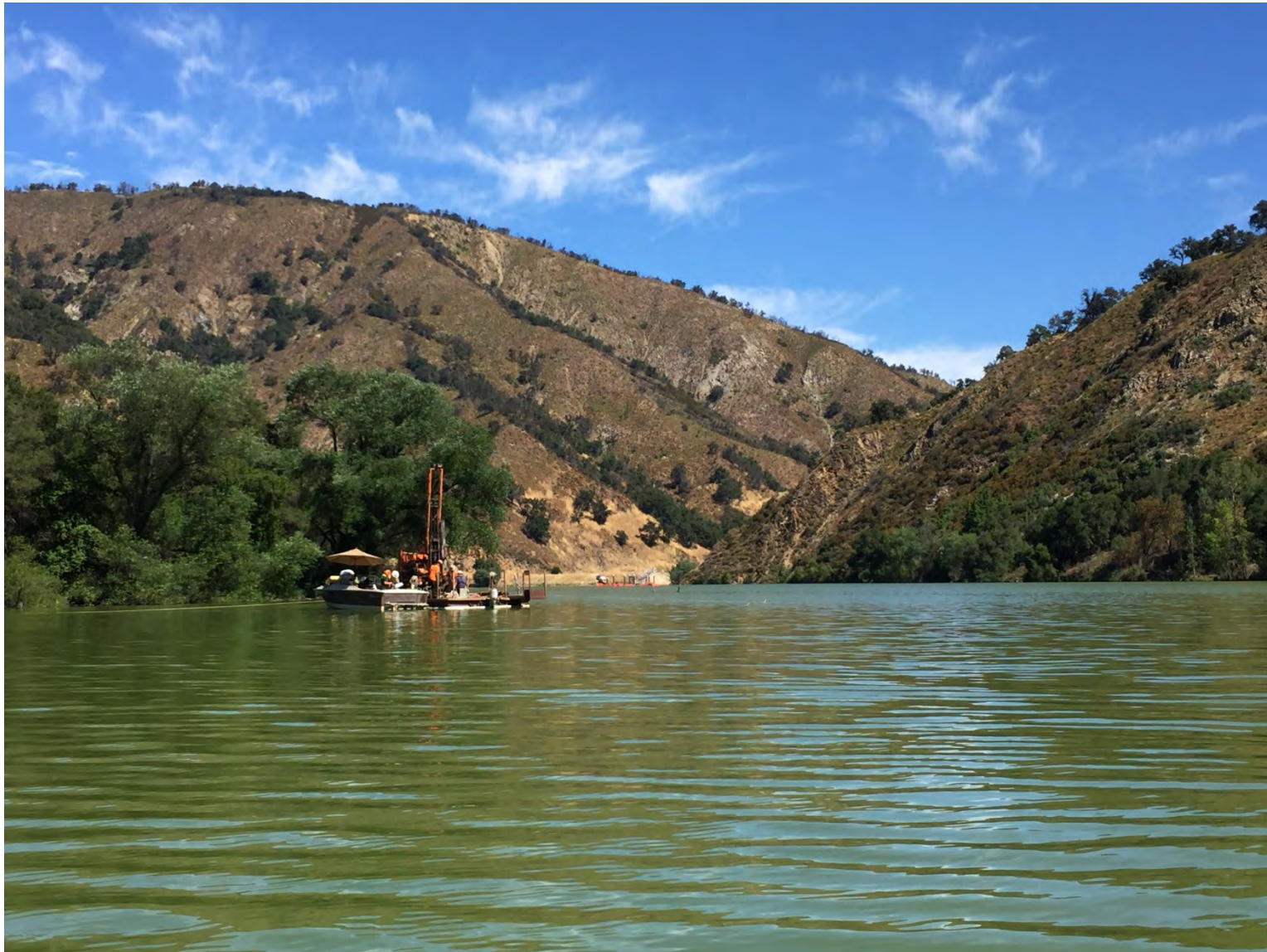
Photo 1. Drill Rig Mounted on Small Platform Barge
