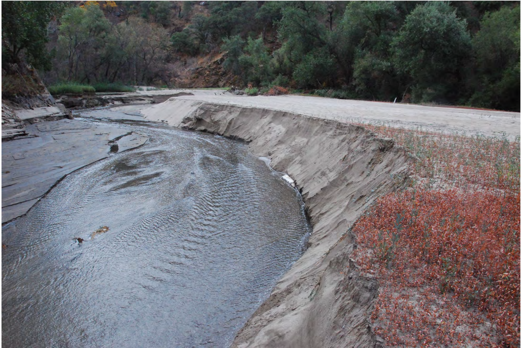
Photo 11. Recently eroded upstream sediment, November, 2017
