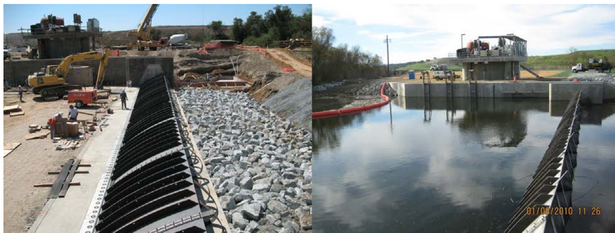
Figure 2-8 Obermeyer Gate at Salinas River Diversion Facility
