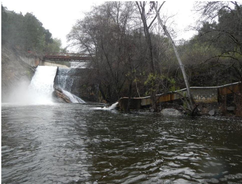
Figure 2-8. Steeppass Fish Ladder below Los Padres Dam, with the Spillway in the Background
