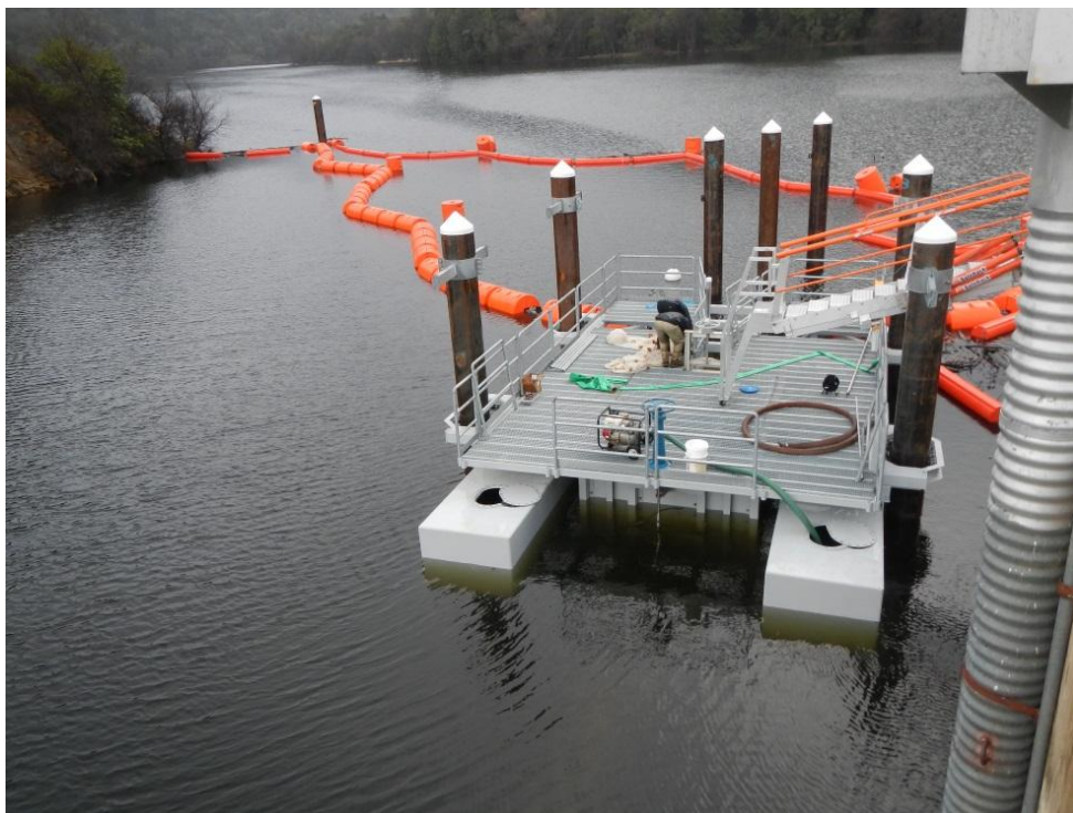
Figure 2-10. Floating Weir Collector for Downstream Fish Passage at Los Padres Dam
