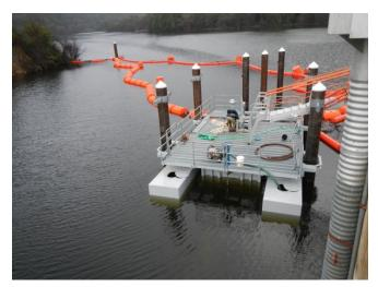
collector (FWC) upstream of the LPD spillway (see photo), which guides downstream-migrating steelhead into a smolt bypass pipe that releases them downstream of LPD. However, data show nearly all downstream-migrating adults use the spillway to navigate LPD; juvenile fish use both the spillway and smolt bypass system.
