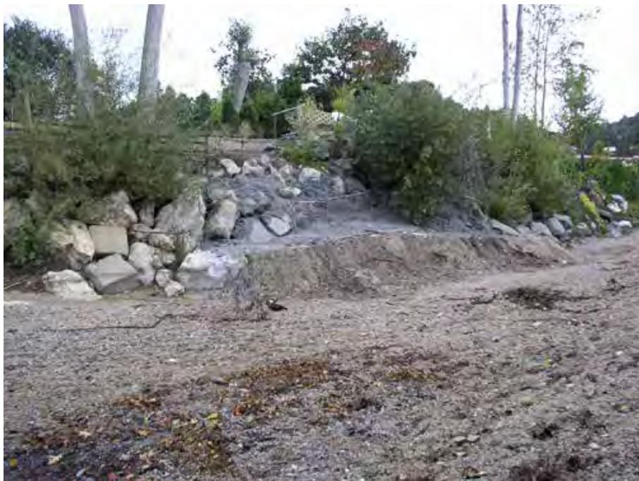
Figure 14. Example of a violation of District rule 124 (cutting riparian vegetation, dumping fill in the active channel, and pumping concrete onto the streambank without a valid permit).
