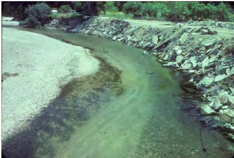
Figure 6. Failing streambank with concrete rubble upstream of Schulte Road Bridge (1982).
