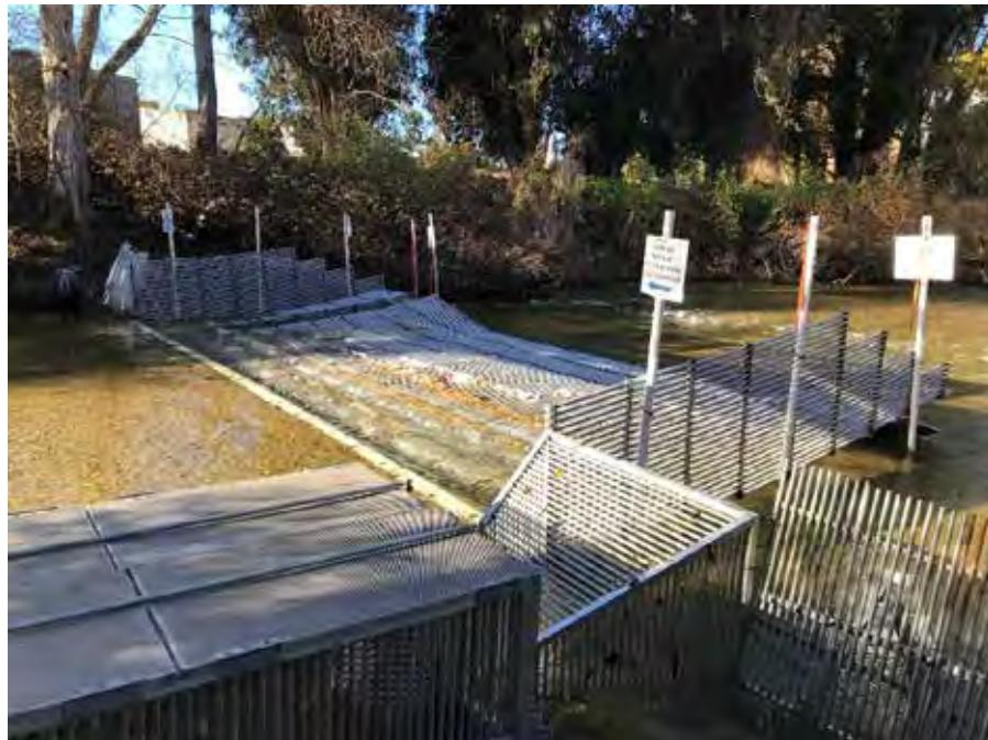
Figure 3. Carmel River Resistance Board Weir (fish counting station).
