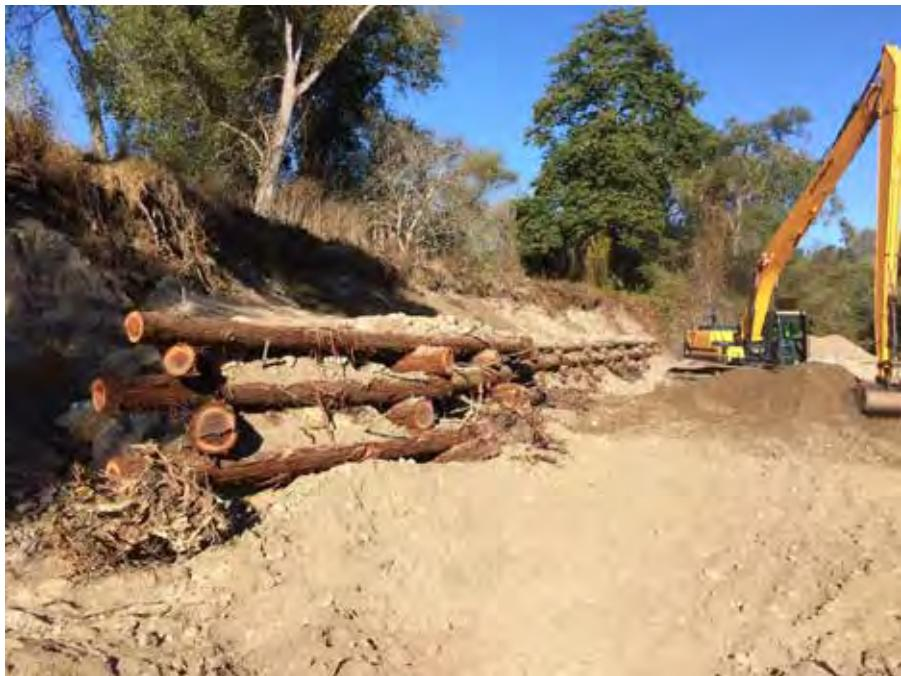
Figure 10. Construction of crib wall at Rancho San Carlos to protect bank from erosion (2018).
