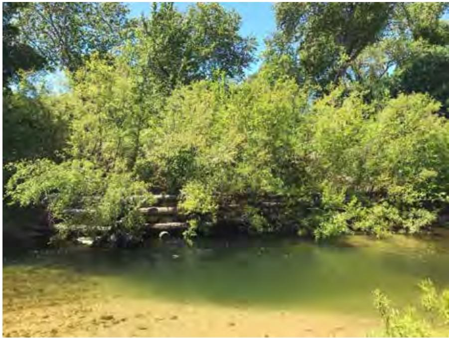
Figure 11. Rancho San Carlos Bank Restoration and Stabilization Project with crib wall and planted willows (2024).
