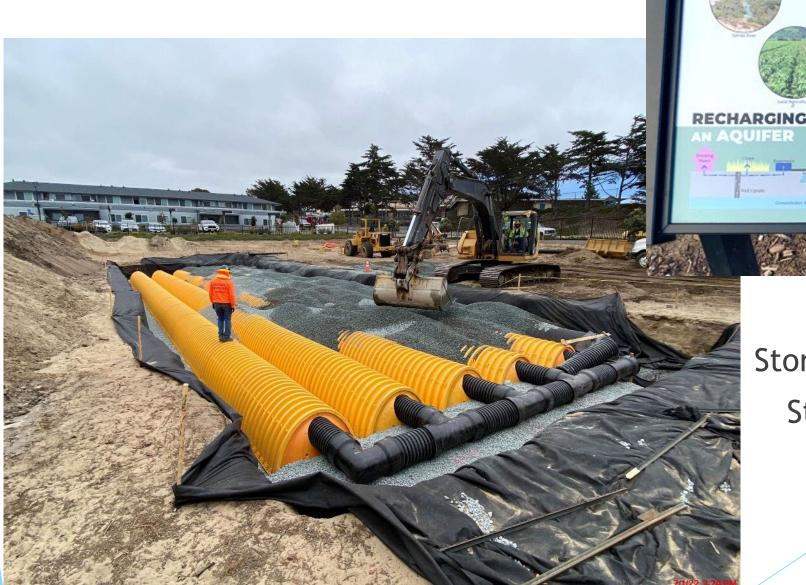
Stormwater Infiltration Chamber
