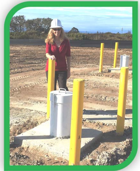
Maureen Hamilton, Project Manager for Injection Well Facilities for the Pure Water Monterey Project (PWM), with test wells. The first PWM injection well was completed in 2017.
