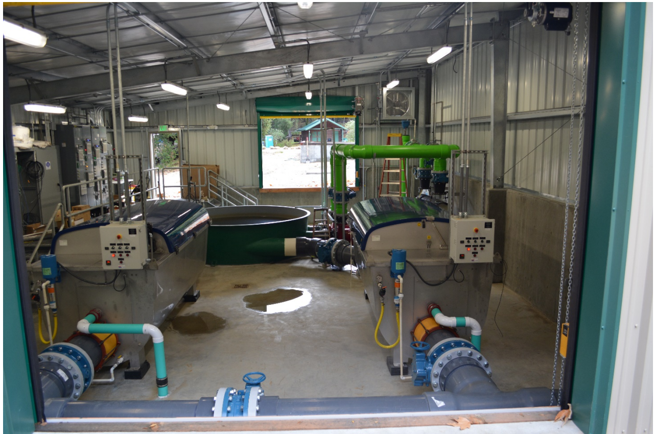
(Photo: Sleepy Hollow Drum Filters)
