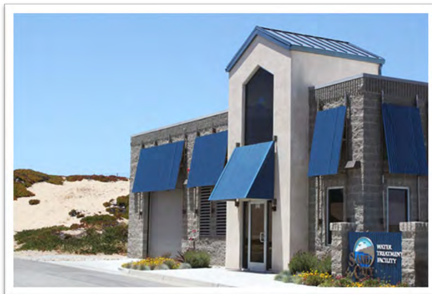
Figure 6-6. Sand City Desalination Plant (Desalination Plant Helps Save a California Coastal Community, 2010).
