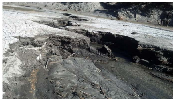
Figure 6-2. Headcutting into the silt and organic deposits in the delta at the head of Los Padres Reservoir.
