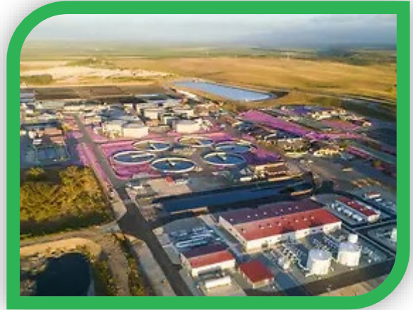
Pure Water Monterey Groundwater Replenishment Project | Recipient of the American Society of Civil Engineers – 2022 Honor Award
