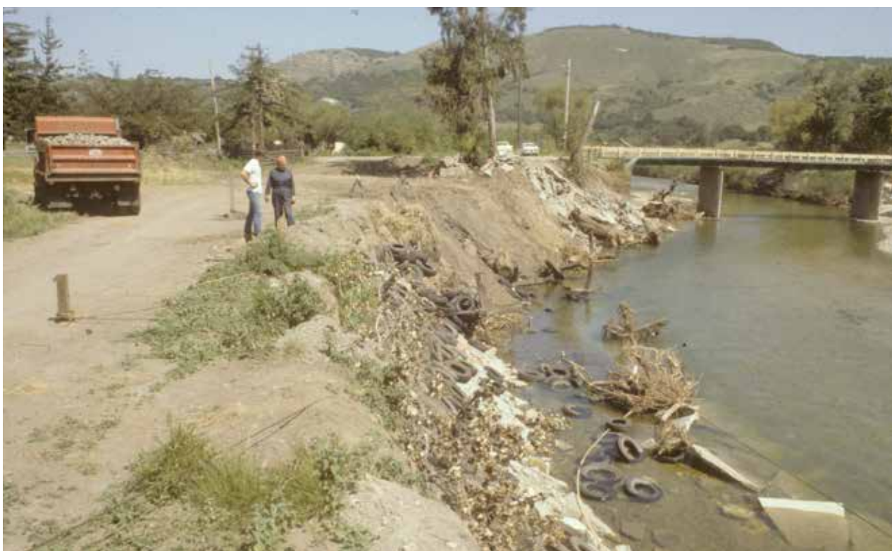
1982 Property owners struggled to prevent erosion by placing old car tires and concrete rubble to try and protect their land from high winter flows. In 1986, MPWMD began work on the Schulte Restoration Project by rebuilding eroded banks near the Schulte Road Bridge. The primary objective of the design was to restore riparian habitat and stabilize the river channel. Image credit: MPWMD.
