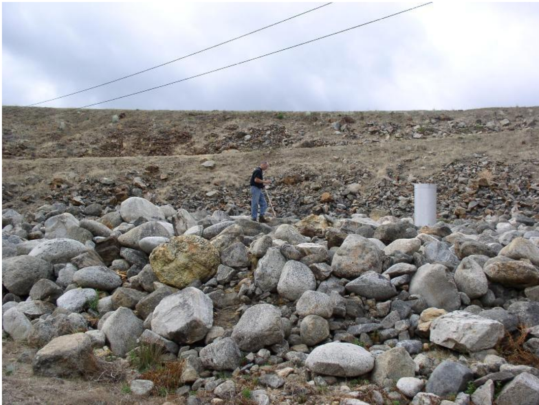
Figure 13 – boulders placed to stabilize downstream face
