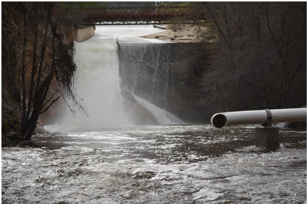
Figure 4 - Looking south to plunge pool and Behavioral Guidance System (BGS) pipe outlet
