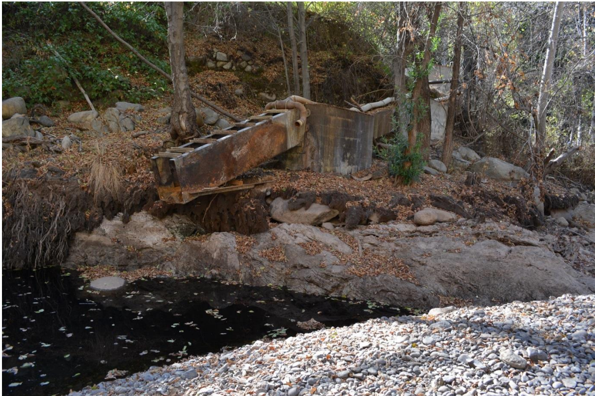
Figure 7 – Existing weir fishway (Denil ladder) entrance in plunge pool
