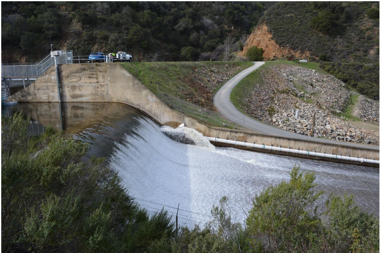
Figure 15 – Looking west at spillway w/BGS anchored to left wall and dam access road in background.
