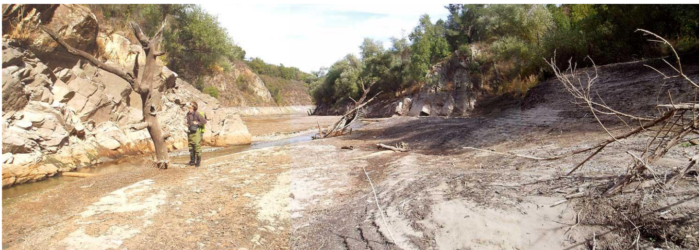
Figure 18 – siltation at upper end of reservoir
