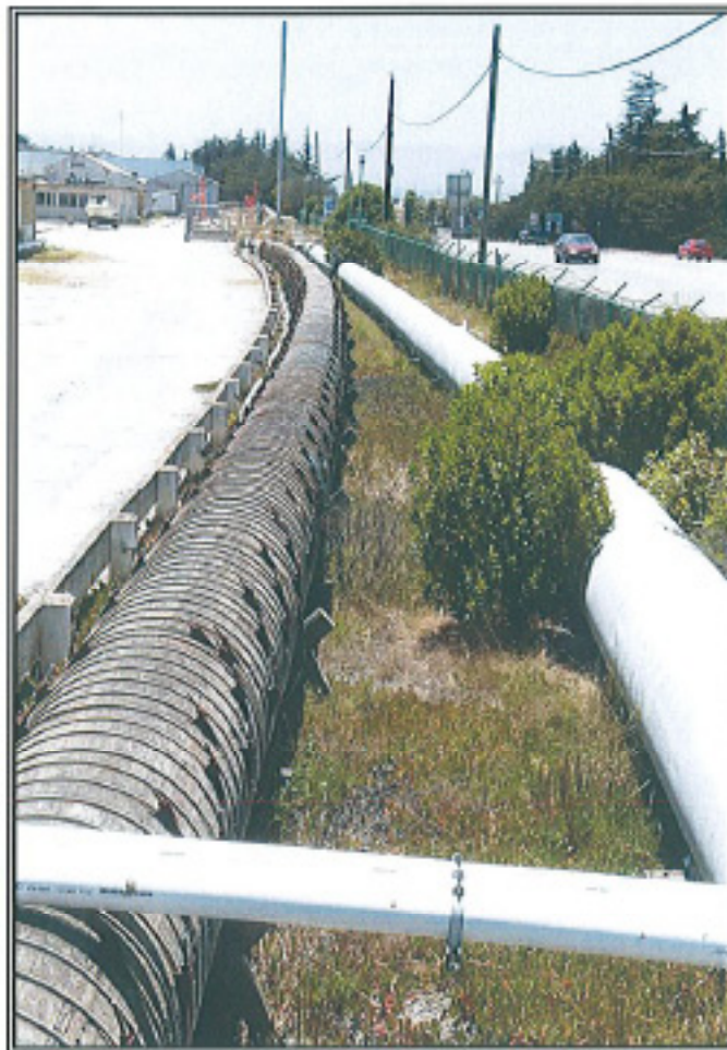
View of intake and outfall pipes running along edge of property next to Highway 1.
