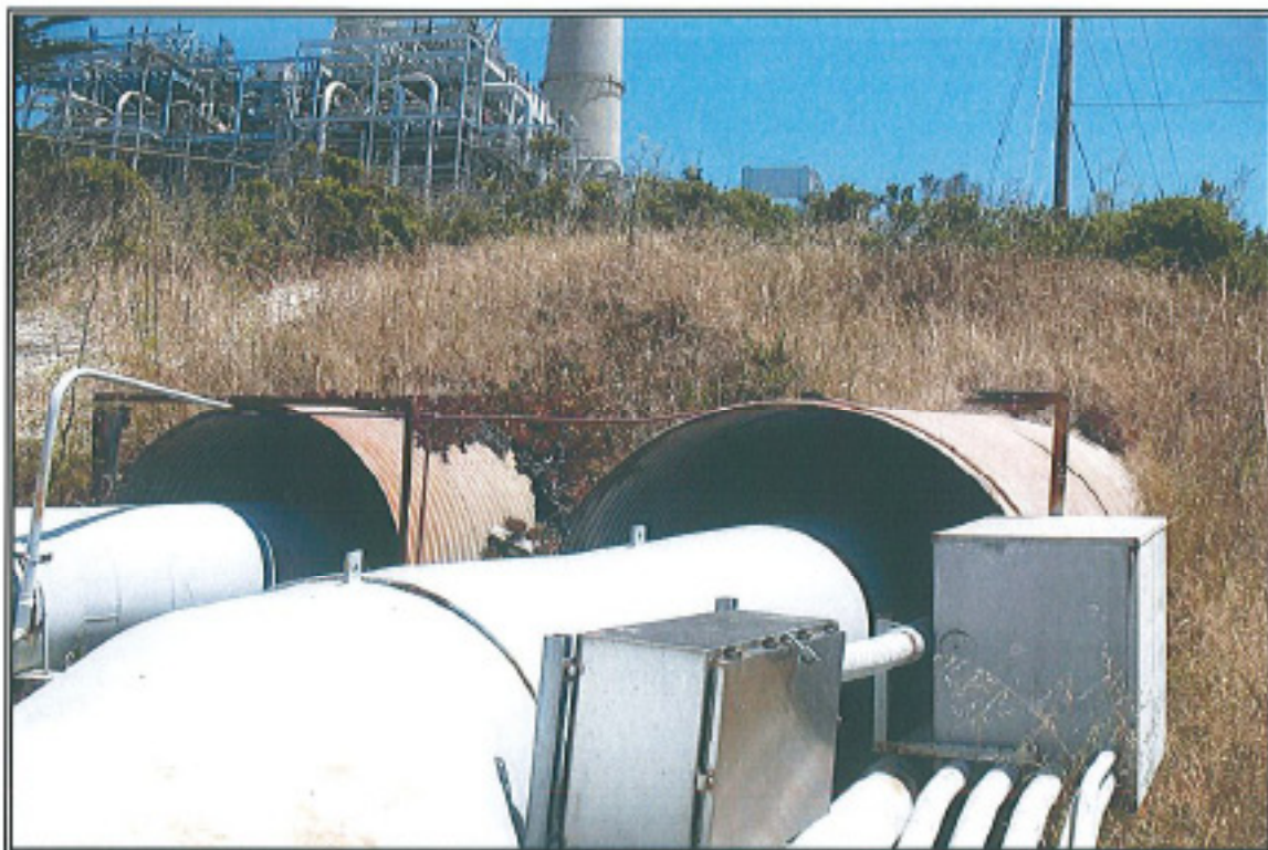
View of intake and outfall pipes emerging from tunnel under Highway 1 on Moss Landing Marina side of highway
