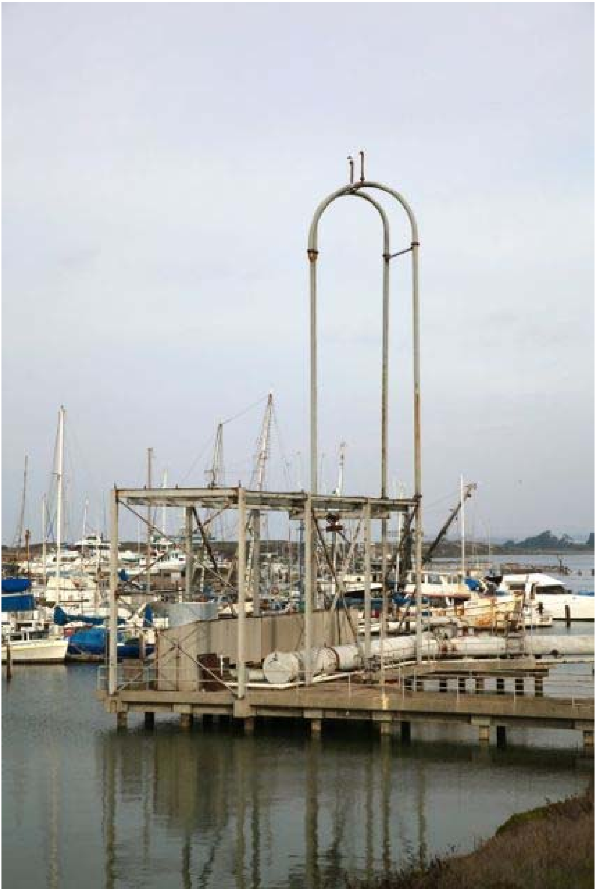
Intake structure at the Moss Landing Harbor
