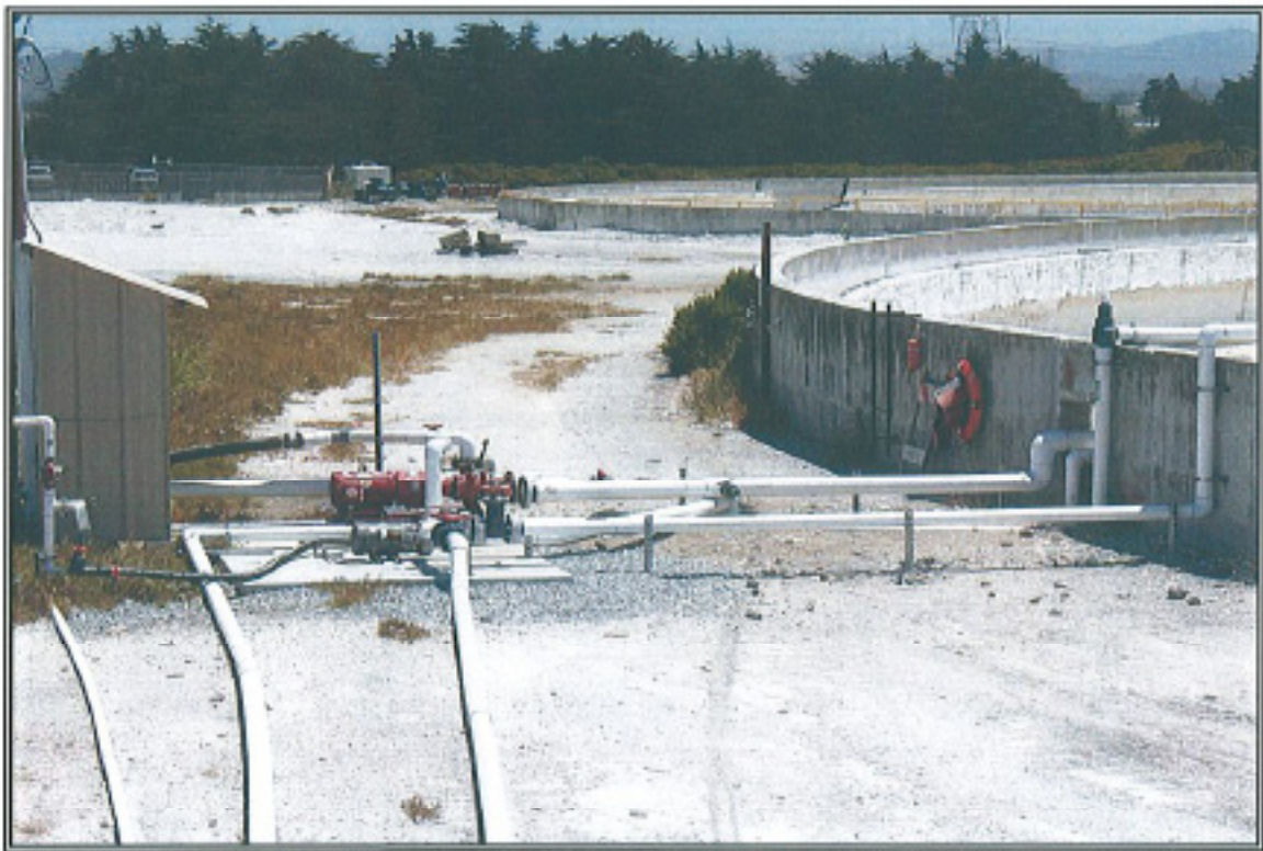
View of typical extensive piping, valves and pumps connecting the various tanks. Note large pipe from under ground going into side of 5-million-gallon tank
