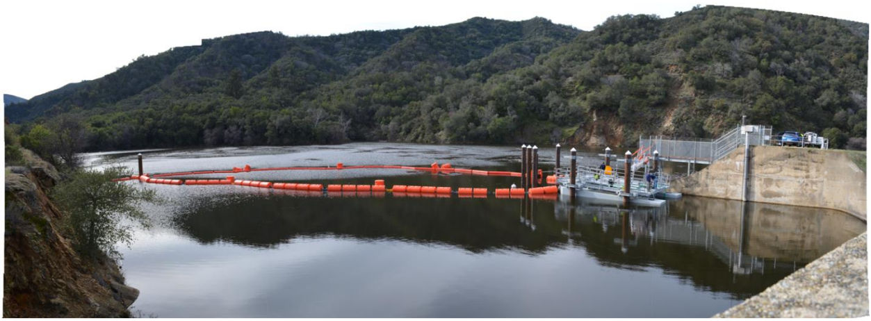
Figure 14 – Behavior Guidance System at dam spillway
