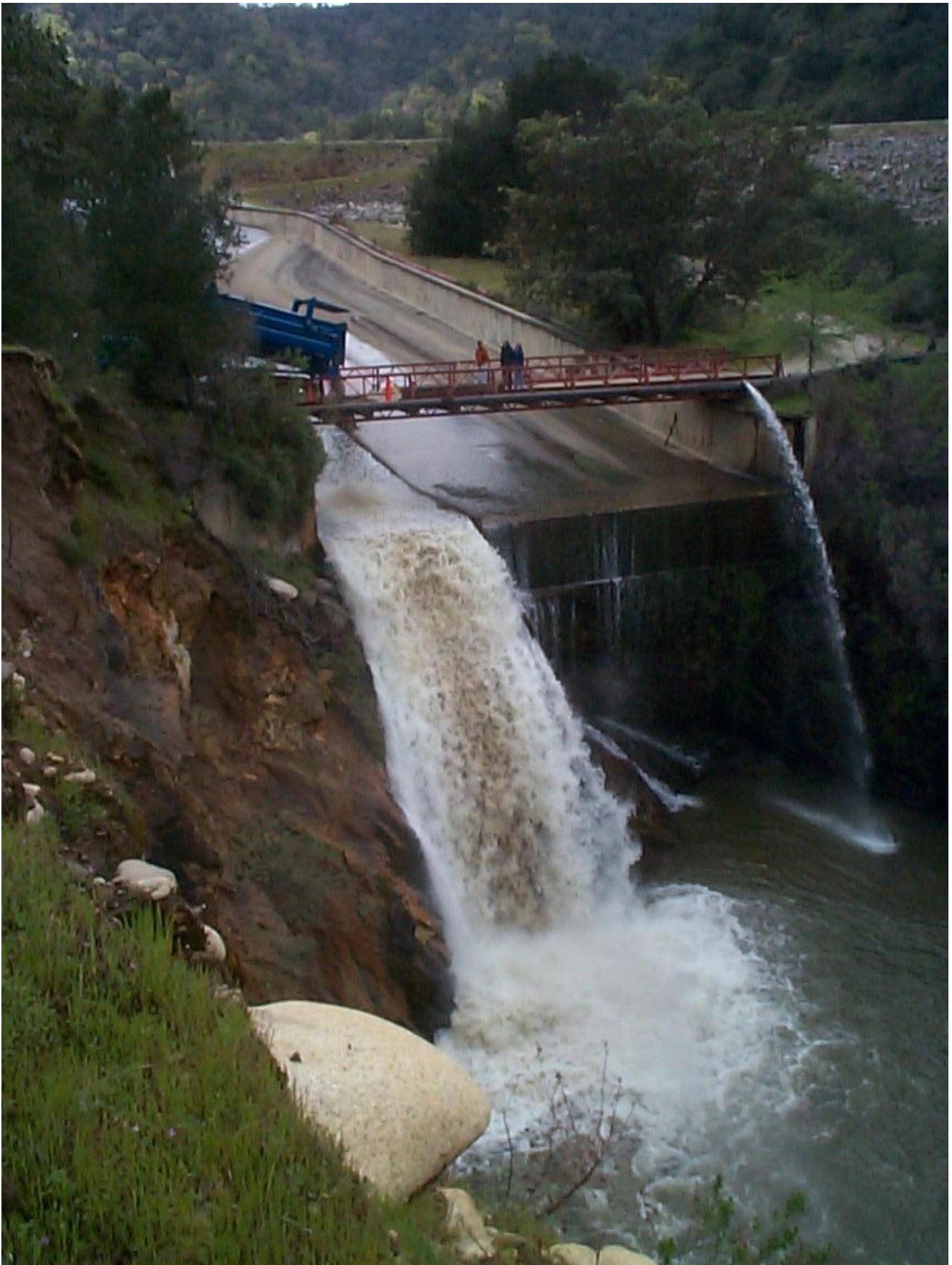
Figure 5 – Bailey Bridge and plunge pool at end of spillway
