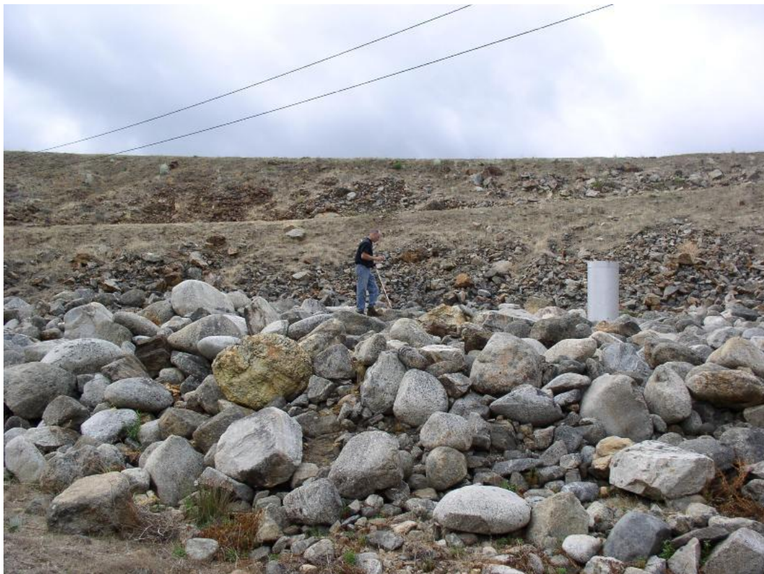
Figure 13 – boulders placed to stabilize downstream face
