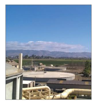
This \$1 million project connected the Pajaro Valley Water Management Agency's (PVWMA) supplemental wells to their existing Recycled Water Coastal Distribution System. The project included 2,800 linear feet of mortar lined and coated welded steel pipe and a static mixing system.
