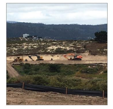
This \$9.4 million project includes the installation of approximately 2,600 linear feet of open-cut pipeline, electrical building construction, percolation basin and deep well, vadose well, and six monitoring wells. SCADA and communication installations at remote sites are also part of the project requiring coordination with partnering agencies including Marina Coast Water District, the City of Seaside, the County of Monterey, and the Fort Ord Redevelopment Agency.
