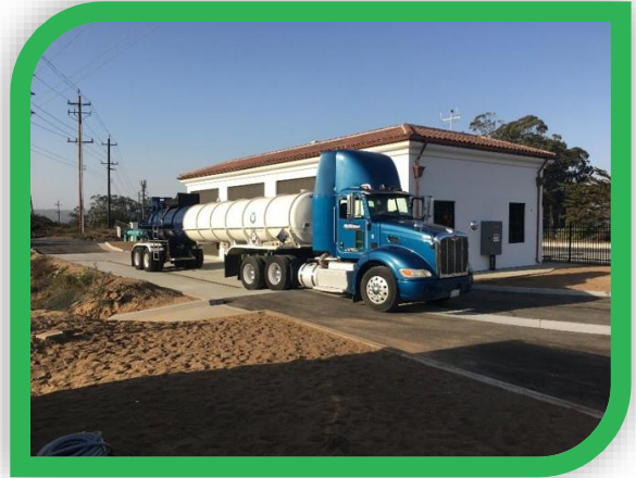
Construction of Santa Margarita Water Treatment Facility was completed in 2020
