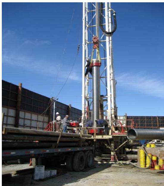
Installation of stainless steel well casing to a depth of 770 feet.
