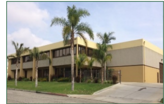
HHCI Headquarters, Riverside, CA
