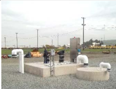
DB Replace Sewer Lift Stations
