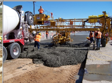
Earthwork, Concrete & Asphalt Paving
