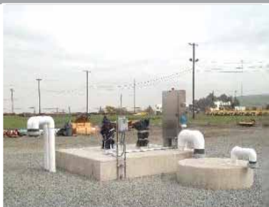
DB Replace Sewer Lift Stations
