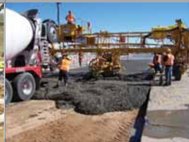
Earthwork, Concrete & Asphalt Paving
