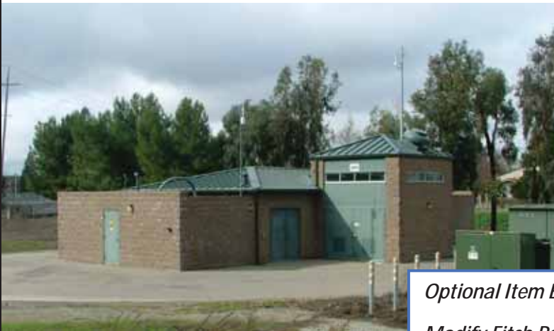
Photo of Mocho ASR Building with CMU Enclosure
