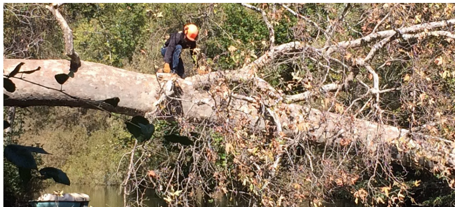
District field crew prepares to remove a large tree that has fallen across the river. The tree creates a hazard that can cause erosion by forcing river flows against streambanks.
