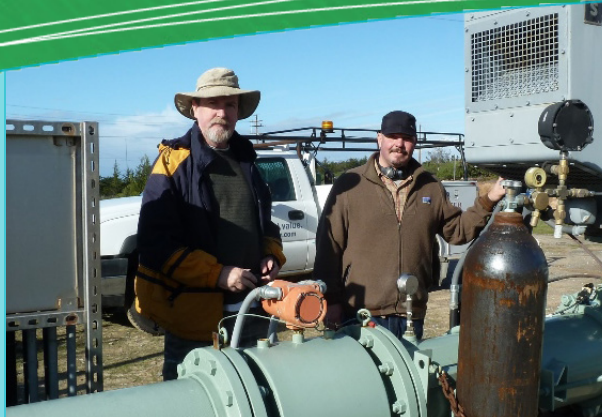
District staff Tom Lindberg and Jon Lear preparing the ASR site for operation. The first week in February, enough water was stored underground daily by the ASR Project to serve 40 homes for a year.
