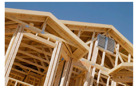
Auxiliary units can be sub-metered as of December 2017. Also, existing multi-family residential sites and common interest developments must retrofit. Rebates are available until January 1, 2019.
