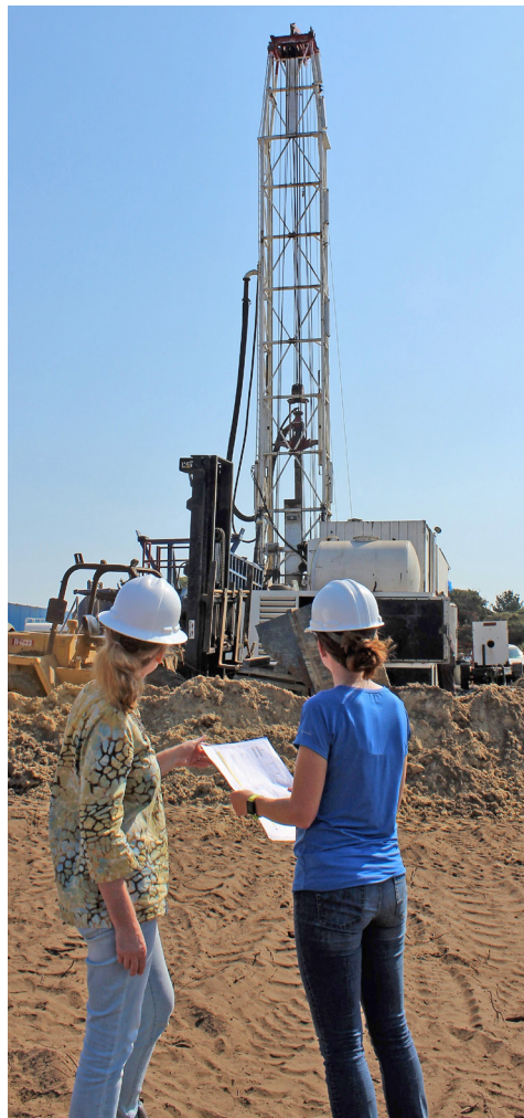
Drilling an injection well. Maureen Hamilton, MPWMD Water Resources Engineer (L), and Amber Ritchie with Todd Groundwater (R) oversee construction. Pure Water Monterey water will be injected underground to mix with existing groundwater before it is delivered to Cal-Am customers.
