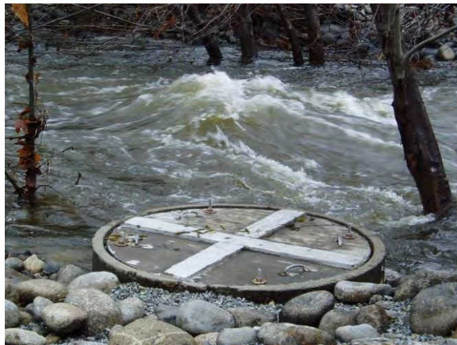
Photograph 6 Intake Pump Housing at 850 cfs
