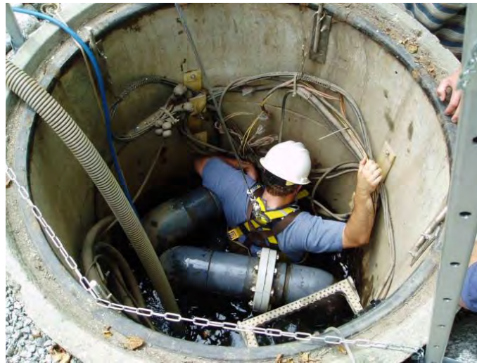
Photograph 5 Intake Pump Housing during Servicing
