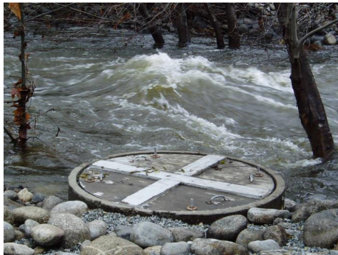
Photograph 6 Intake Pump Housing at 850 cfs
