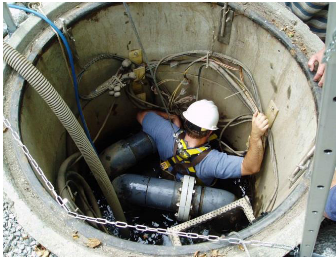
Photograph 5 Intake Pump Housing during Servicing
