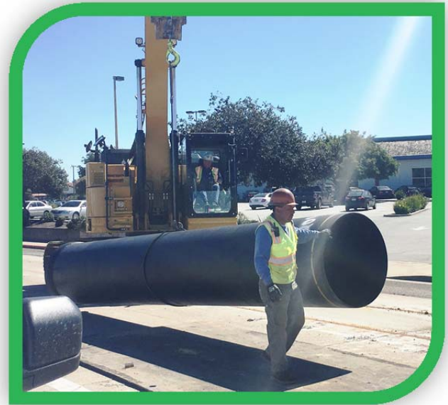
New Monterey Pipeline under construction to facilitate distribution of water from the Pure Water Monterey project, and transmit excess Carmel River water to ASR wells in the winter.
