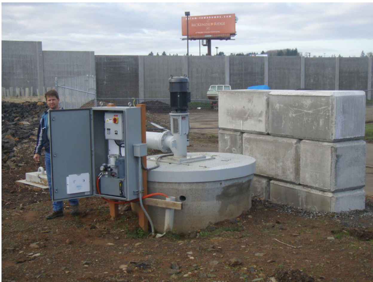
Image 3- Example of pump motor and electrical supply raised out of wet well to improve access.
