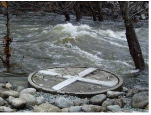
Existing pumps are located next to the river deep inside a concrete caisson (above and left) that is inaccessible at high flows. The existing drum screen (at right) is subject to clogging from silt, sand, and debris.
