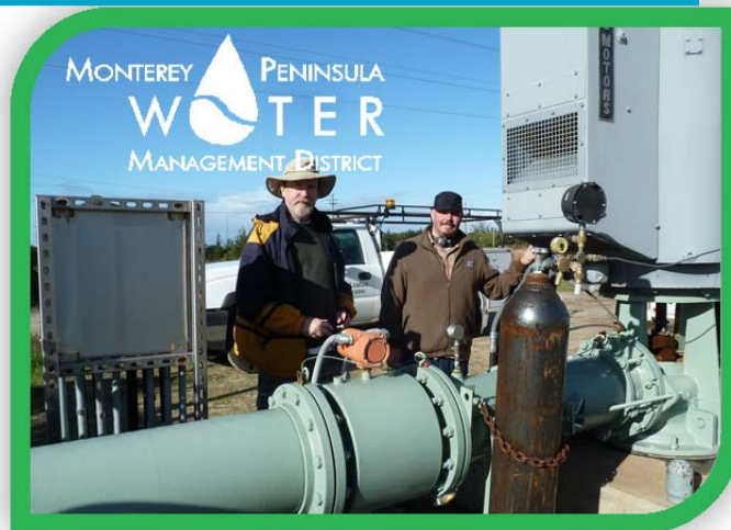
The Water Management District's Aquifer Storage and Recovery project site.
