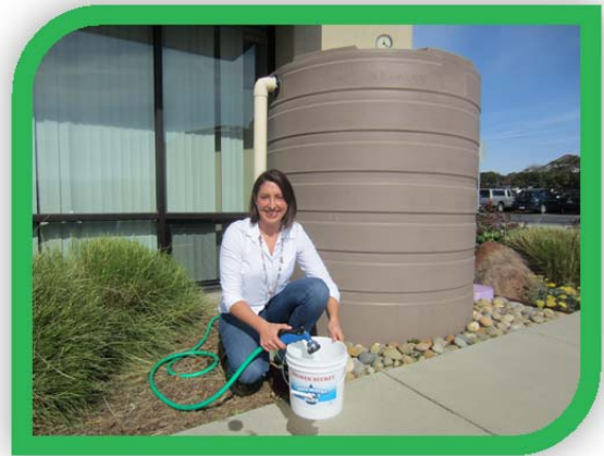
The District offered training on rainwater harvesting methods such as installation of cisterns.
