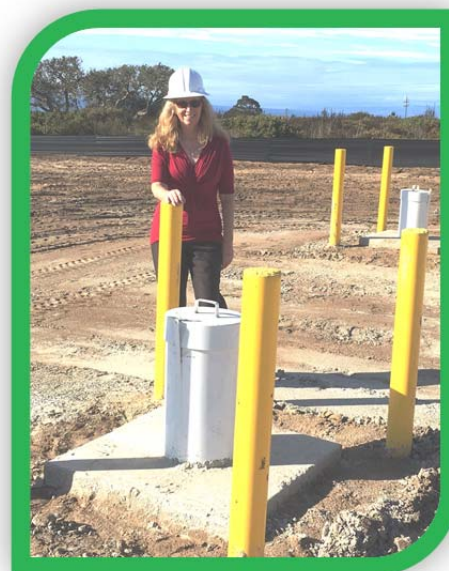
Maureen Hamilton, Project Manager for Injection Well Facilities for the Pure Water Monterey Project (PWM), with test wells. The first PWM injection well was completed in 2017.
