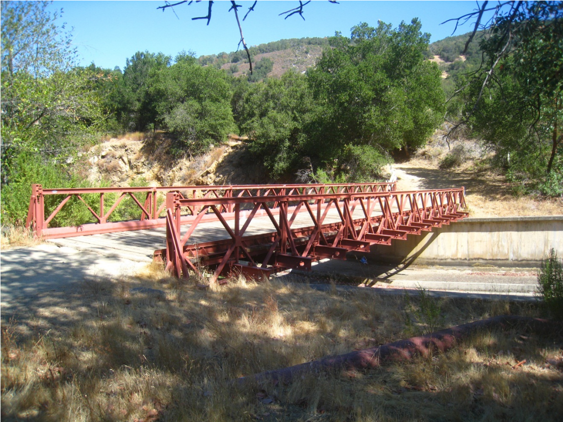
Spillway bridge (September 14, 2012)
