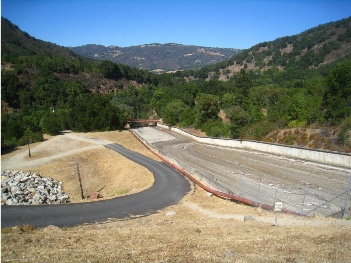
Dam access road (September 14, 2012)
