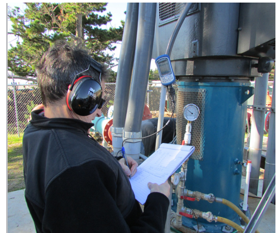
Joe Oliver, MPWMD Water Resources Manager, collects data at ASR Well # 3. Enough water to serve 1,450 homes for a year has been stored for later use by the ASR project.
