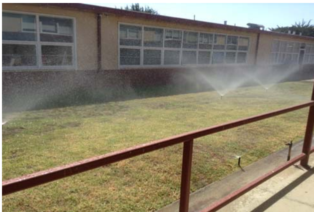
High Water-Use Inefficient Fixed Spray Sprinklers
